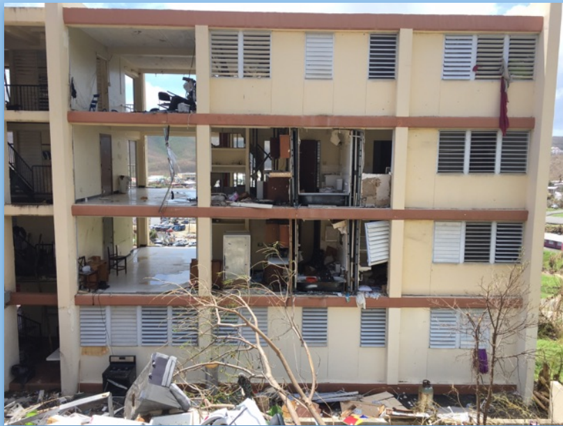
HUD OIG special agents conducted a preliminary damage assessment of the Virgin Islands Housing Authority, Estate Tutu Apartments, St. Thomas, U.S. Virgin Islands. This image displays damage post-Hurricane Irma and pre Hurricane Maria.
