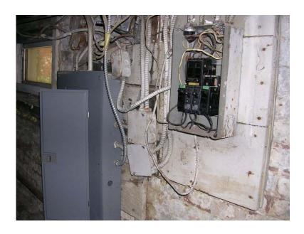
Exposed wiring on an electrical panel found during a May 5, 2006, inspection.
