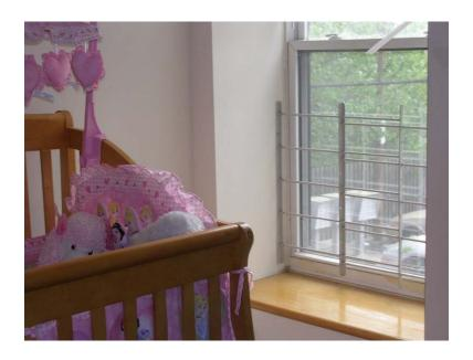
Many units contained egress deficiencies. This unit inspected on May 8, 2006 contained security bars, which could not be opened by those present at the inspection, for all windows located in this room.
