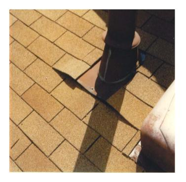
The roof is bowing on the "B" building indicating that sheathing needs to be replaced. Some shingles were improperly installed and are not laying flat on the roof surface. Vinyl siding installation is incomplete.
