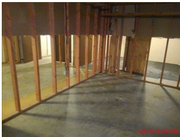
Photo showing that drywall has been removed.
