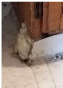
Foam used to try to stop the mice ingress at CARA
