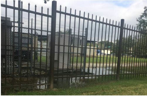
Raw sewage present on property at Texas Coppertree Village
