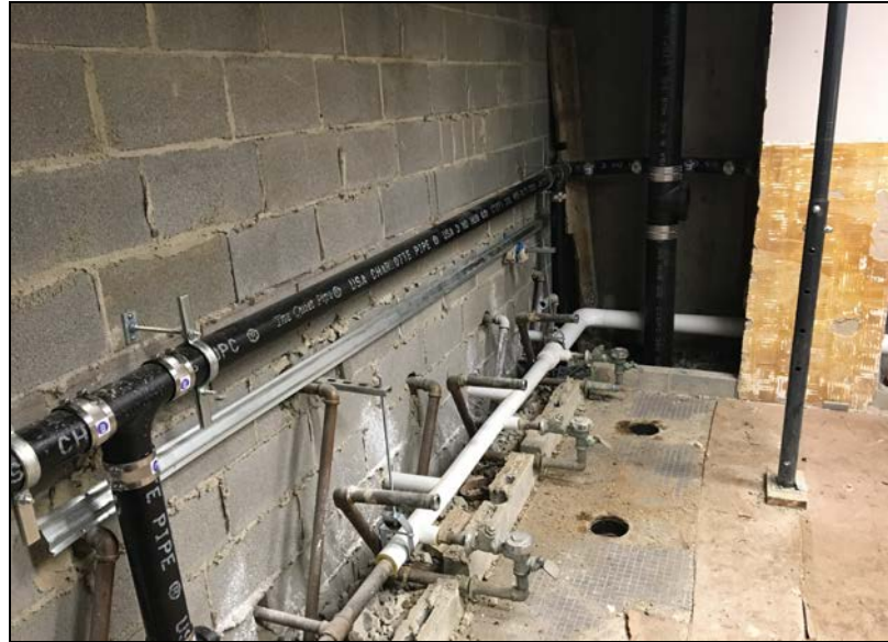
Photo of sanitary piping replaced in restroom facilities located on the fifth floor of the Weaver Building. Photo taken August 21, 2018.
