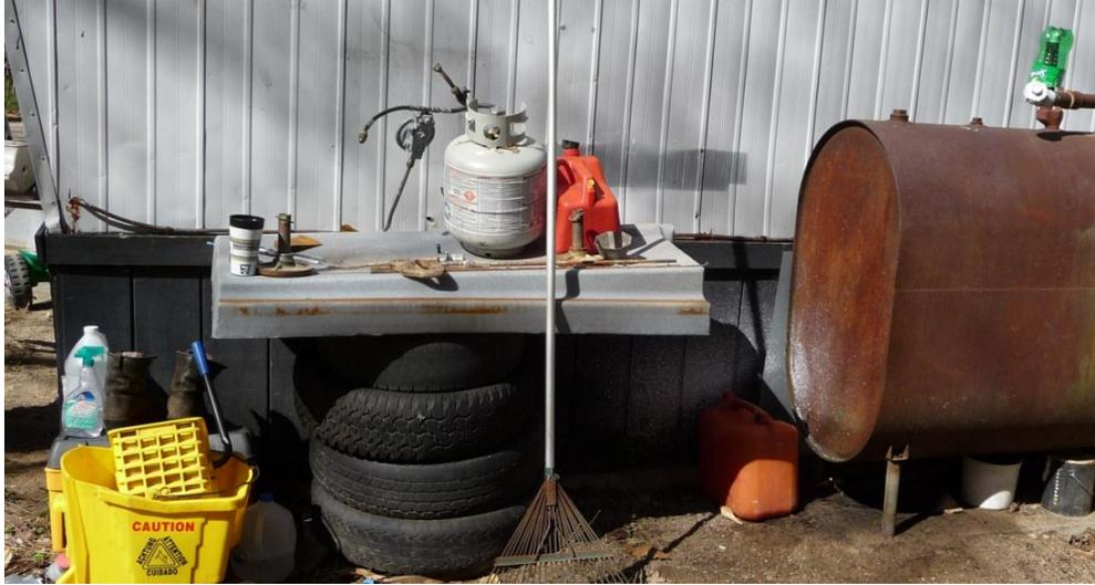
The picture above shows a 5-gallon portable propane tank located at the rear of the unit, which was connected to the kitchen stove. The propane tank was on top of a flat plastic container supported by four rubber vehicle tires near a gas can and an oil tank, which was a potential fire hazard.
