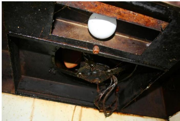
The picture above shows a stove vent hood motor that did not work and was covered in grease, which was a preexisting condition as well as a fire hazard.
