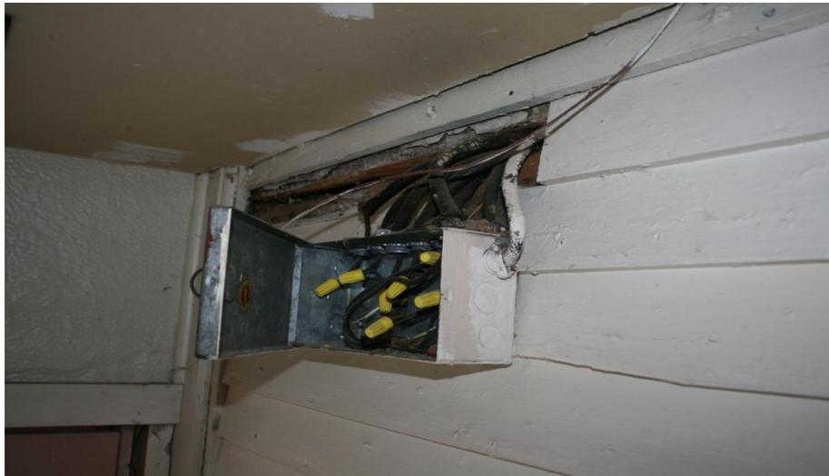
The picture above shows a preexisting electrical issue of wiring coming from a hole in the wall into a junction box that was not secured, exposing more wire in the foyer-entrance to a unit.
