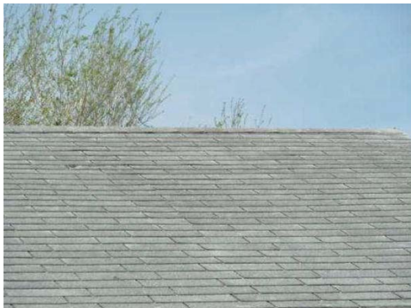
Figure 2: Sample home 1. The inspection stated that wind damaged the roof covering. This roof picture did not identify the Hurricane Dolly wind damage.
