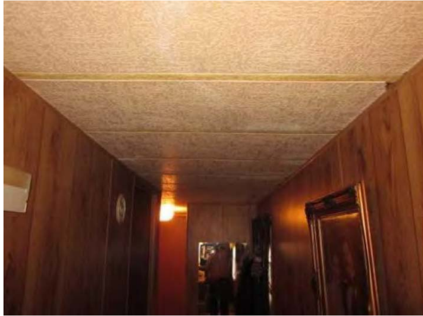
Figure 5: Sample home 44. The inspection stated that Hurricane Dolly damaged the interior ceiling and walls; however, the pictures did not identify the hurricane damage. 6
