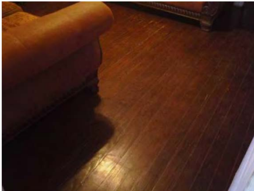
Figure 4: Sample home 18. This picture of the flooring in the living room did not show hurricane storm surge damage. The file did not contain pictures that showed storm surge damage to the flooring or walls.
