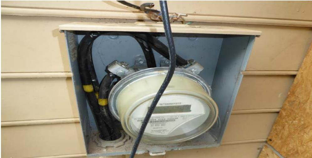
The picture above shows that the cover on an electric meter box is missing the seal and can be easily opened, exposing electrical contacts and creating an electrical hazard such as shock.
