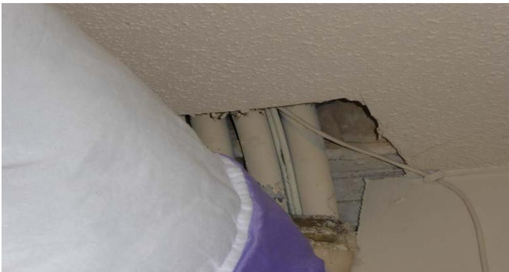
The picture above shows a large hole in a closet ceiling through which pipes are passing. The large hole allows for vermin, dust, and air infiltration.
