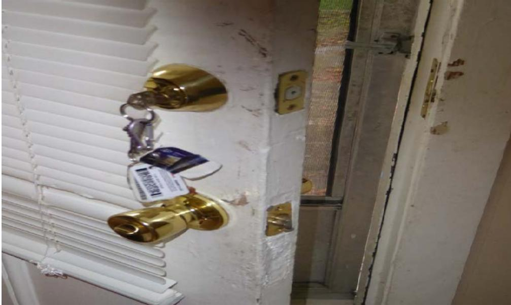
The picture above shows a keyed deadbolt lock on the kitchen exit door. If the tenant cannot find the key, exit would be blocked in case of emergency.
