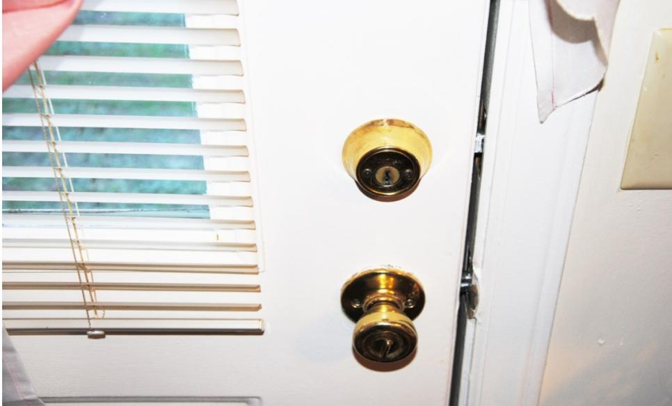
The picture above shows a keyed deadbolt lock on the kitchen exit door. If the tenant could not find the key, the exit would be blocked in case of emergency.
