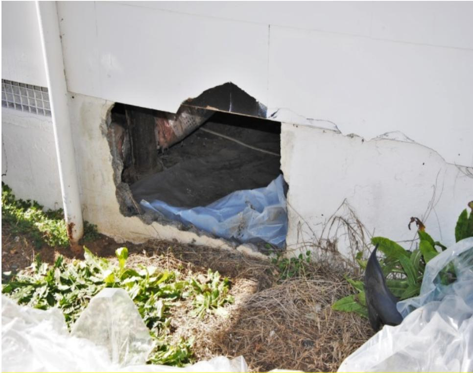
The picture above shows a large hole in the foundation of the property, allowing water, air, and insect infiltration.
