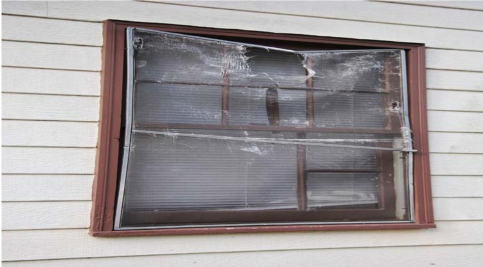
This picture shows a bent frame and torn screen on a window. The tenant could not open the window without letting insects and debris into the house.
