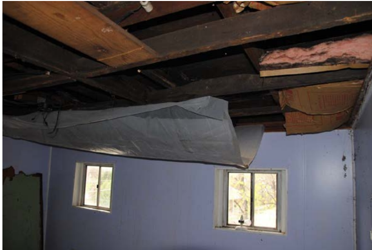
Inspection #46: Plastic sheets were used to catch roof leaks in the attic and drain into scattered buckets. The Authority did not identify this violation during its February 3, 2015, inspection.
