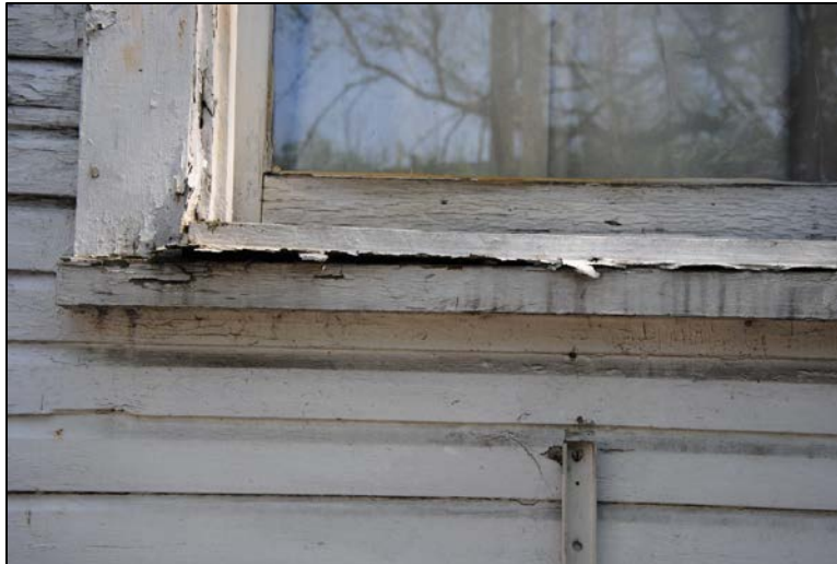
Inspection #16: Window sill components were deteriorating, separating, and allowing moisture into the wall. The Authority did not identify this violation during its January 15, 2015, inspection.
