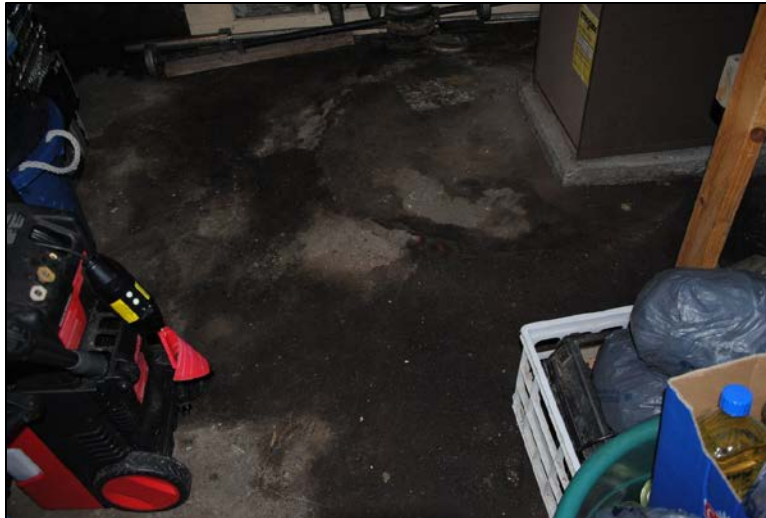
Inspection #2: The floor in the basement was wet, and the basement had a musty odor due to a leak in the foundation. The Authority did not identify this violation during its November 21, 2014, inspection.
