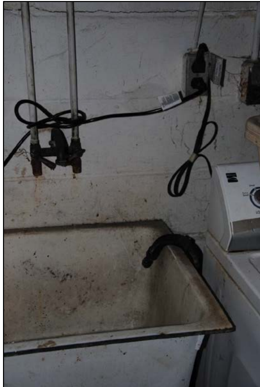
Inspection #21: An outlet on a basement wall was within 3 feet of a water source, and it was not a GFCI (ground fault circuit interrupter). The Authority did not identify this violation during its November 17, 2014, inspection.
