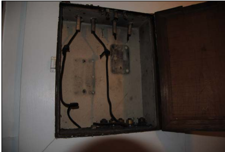
Inspection #51: Live electric wires exposed in an unsecured cabinet, recessed in the wall of the stairway's second floor. The Authority did not identify this violation during its February 2, 2015, inspection.
