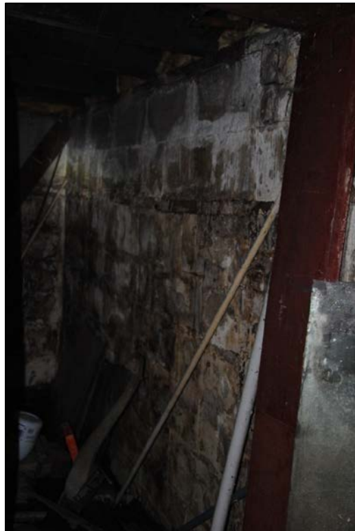
Inspection #12: The walls in the basement showed signs of mold due to a water leak. The Authority did not identify this violation during its November 18, 2014, inspection.
