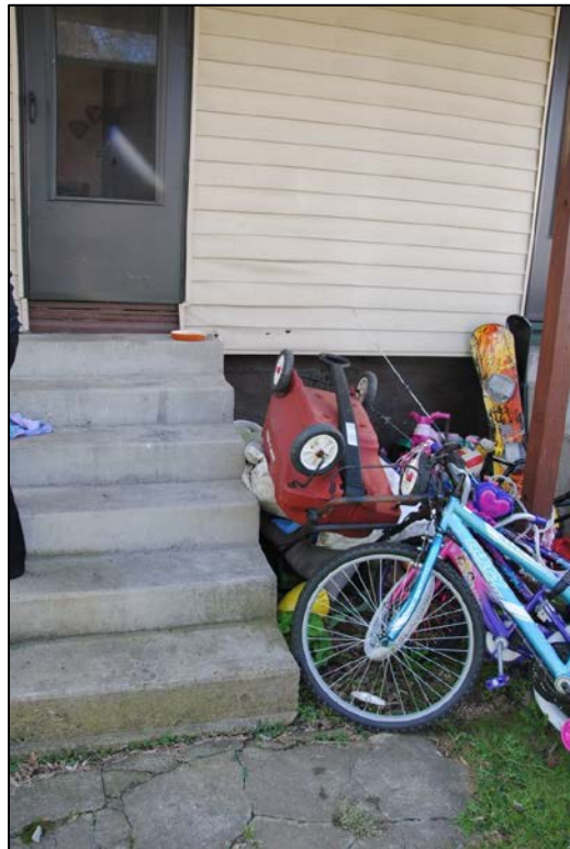
Inspection #17: The rear stairway had an open side that was higher than 30 inches, requiring a guardrail. The Authority did not identify this violation during its December 18, 2014, inspection.
