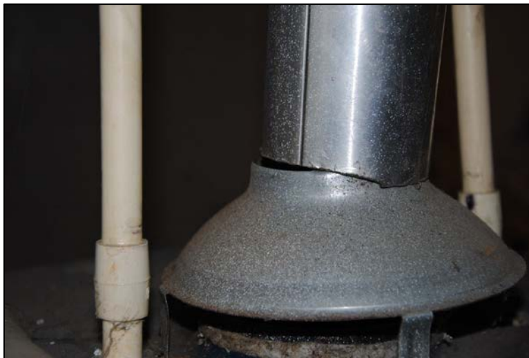
Inspection #33: The water heater flue was not well connected to the draft hood. The Authority did not identify this violation during its November 17, 2014, inspection.
