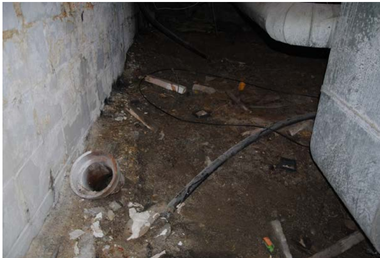
Inspection #71: Exposed sewer line was stuffed with a rag. The line must be permanently capped to eliminate sewer gas. The furnace was in the same location. The Authority did not identify this violation during its December 4, 2014, inspection.
