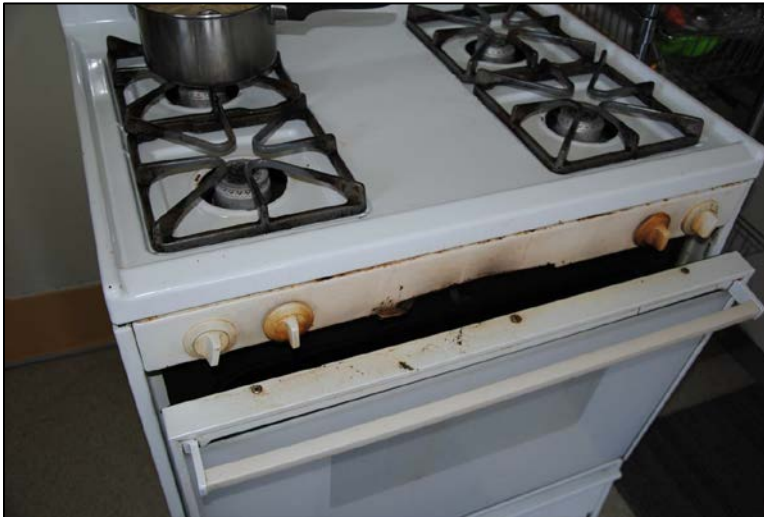
Inspection #50: The kitchen range oven door did not stay closed and scorched the exterior of the range. The Authority did not identify this violation during its November 21, 2014, inspection.
