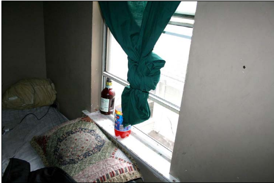
Inspection #64: The upper window sash fell. The Commission did not identify this violation during its February 1, 2016, inspection.
