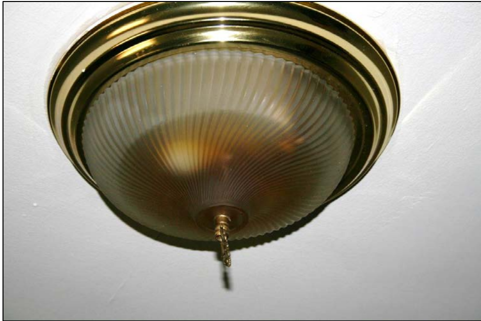
Inspection #48: The light globe in a bedroom was partially filled with water. The Commission did not identify this violation during its December 16, 2015, inspection.
