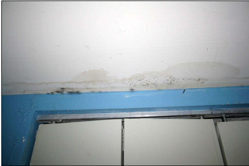
Inspection #3: Mold or mildew was located in the bedroom ceiling above the closet. The Commission did not identify this violation during its December 31, 2015, inspection.
