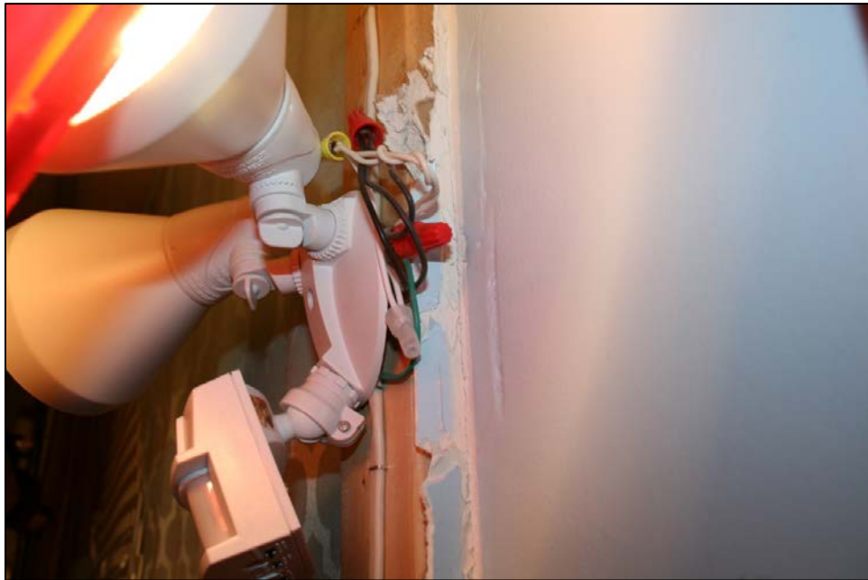
Inspection #56: The motion light was not properly installed and had exposed wiring. This light was located in a garage that the tenant used as a play room. The Commission did not identify this violation during its February 25, 2016, inspection.
