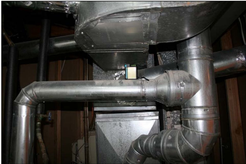
Inspection #7: The vent on the hot water heater had a negative slope, which prohibited gases from venting properly. The Commission did not identify this violation during its December 16, 2015, inspection.
