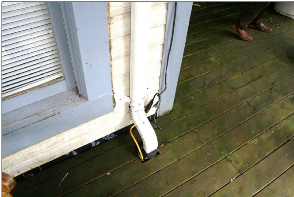
Inspection #44: An extension cord ran from the outlet to the sump pump to provide power. The electrical connection should be weather proof and properly installed. The Commission did not identify this violation during its December 23, 2015, inspection.
