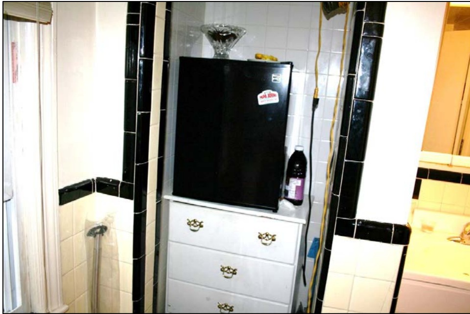
Inspection #37: An electrical cord ran along the floor to the shower to provide power to a refrigerator, and the cord was wrapped around the shower head. The Commission did not identify this violation during its December 15, 2015, inspection.
