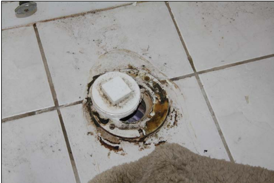
Inspection #58: The toilet was missing, and there was an open sewer pipe. The Commission did not identify this violation during its January 26, 2016, inspection.
