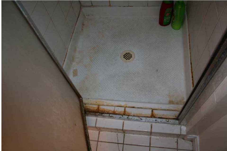
Inspection #58: Mold or mildew was located in the shower on the second floor. The Commission did not identify this violation during its January 26, 2016, inspection.
