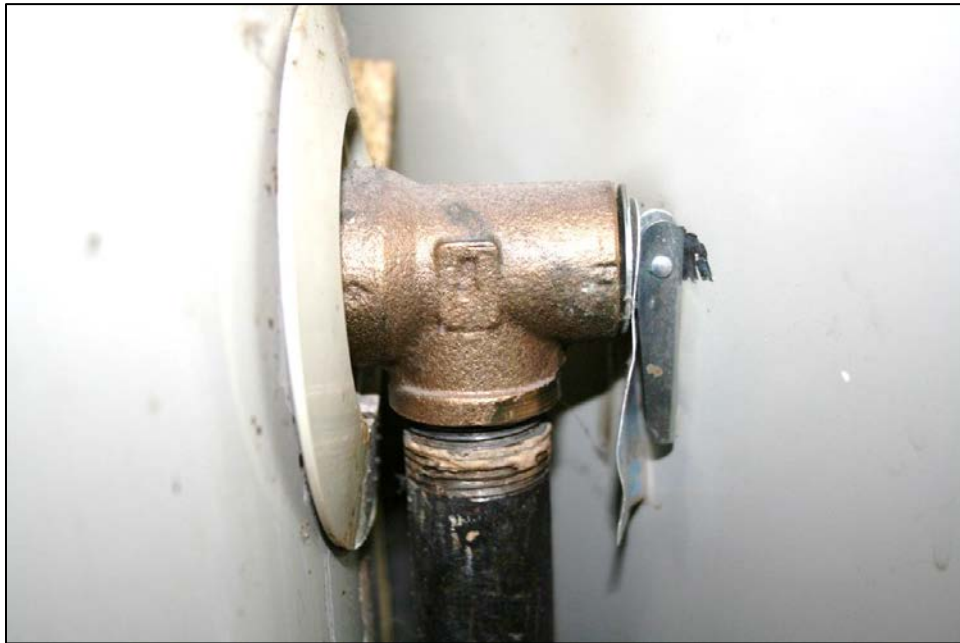
Inspection #70: The temperature and pressure relief valve on the hot water heater was touching the wall and could not be opened, which could result in an explosion. The Commission did not identify this violation during its February 12, 2016, inspection.
