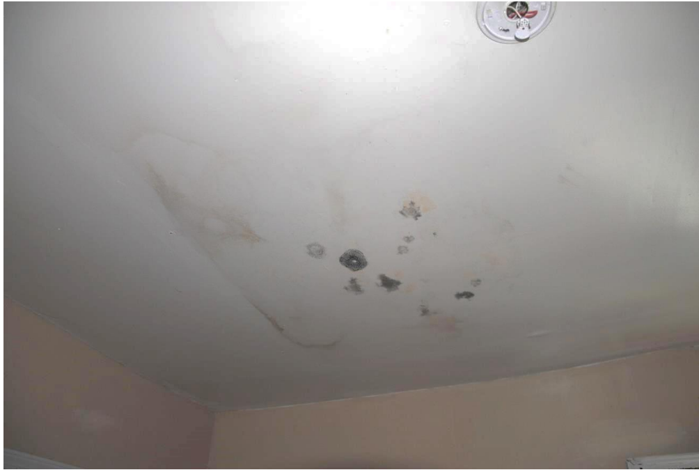
The photo above shows possible mold that had developed on a bedroom ceiling likely due to a leak in the deteriorated roof.
