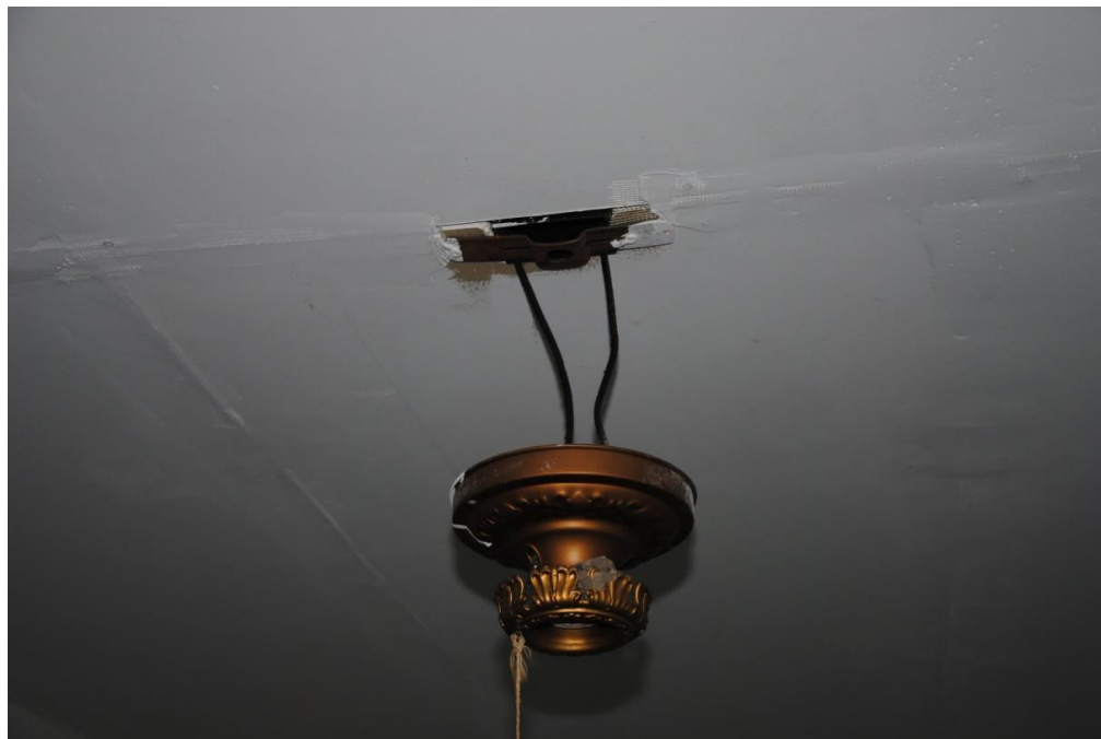
The photo above shows one of three light fixtures hanging from electrical wire on a unit's attic ceiling, resulting in exposed electrical contacts being accessible to the tenants.
