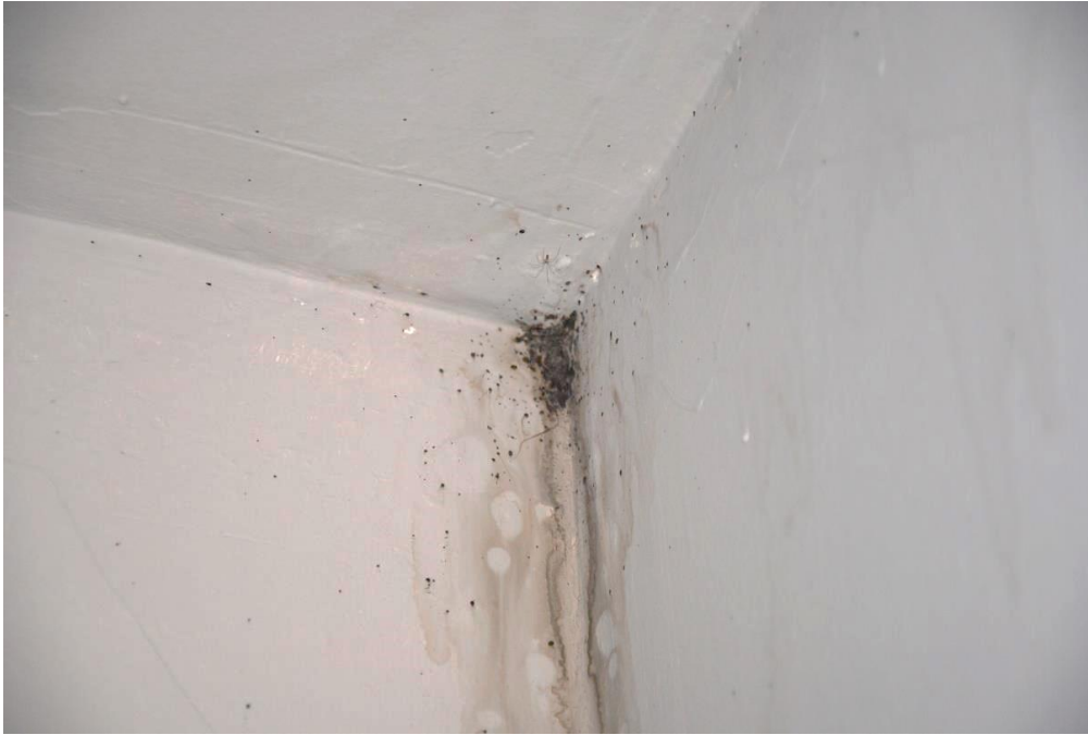
The photo above shows the remnants of an infestation in the corner of a unit's bedroom.
