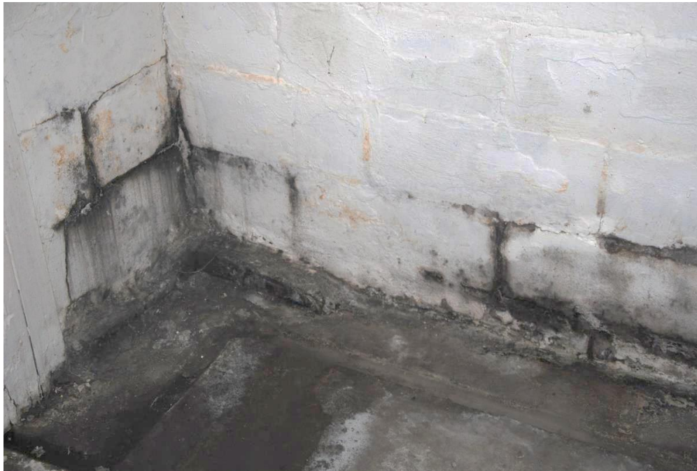
The photo above shows water and possible mold on a basement floor and walls due to leaks in the foundation.
