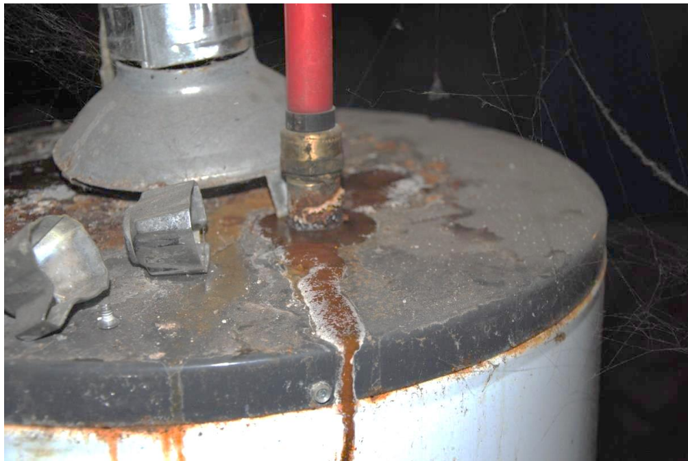
The photo above shows a rusting and leaking water pipe on a unit's water heater that could fail and cause the basement floor to flood.
