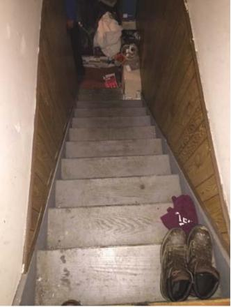
Inspection 5: The handrail in the basement stairway was missing. The Authority did not identify this violation during its November 4, 2016, inspection.
