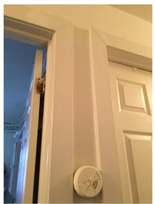
Inspection 38: The smoke detector in the 2<sup>nd</sup> floor hall was installed too low on the wall. The Authority did not identify this violation during its November 14, 2016, inspection.
