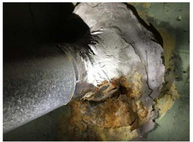
Inspection 49: The boiler flue was corroded next to the chimney and had a hole in it. The Authority did not identify this violation during its November 1, 2016, inspection.
