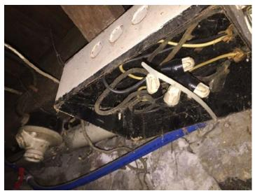
Inspection 50: An old fuse box on the basement ceiling was used as a junction box but had no cover plate. The Authority did not identify this violation during its December 27, 2016, inspection.
