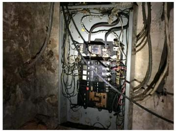
Inspection 32: An unsecured electric panel on a basement wall had no cover on it. The Authority did not identify this violation during its January 17, 2017, inspection.
