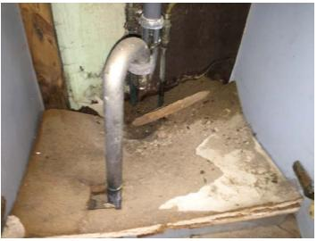
Inspection 51: The floor in the basement bathroom vanity was moisture damaged and collapsed. The Authority did not identify this violation during its November 28, 2016, inspection.
