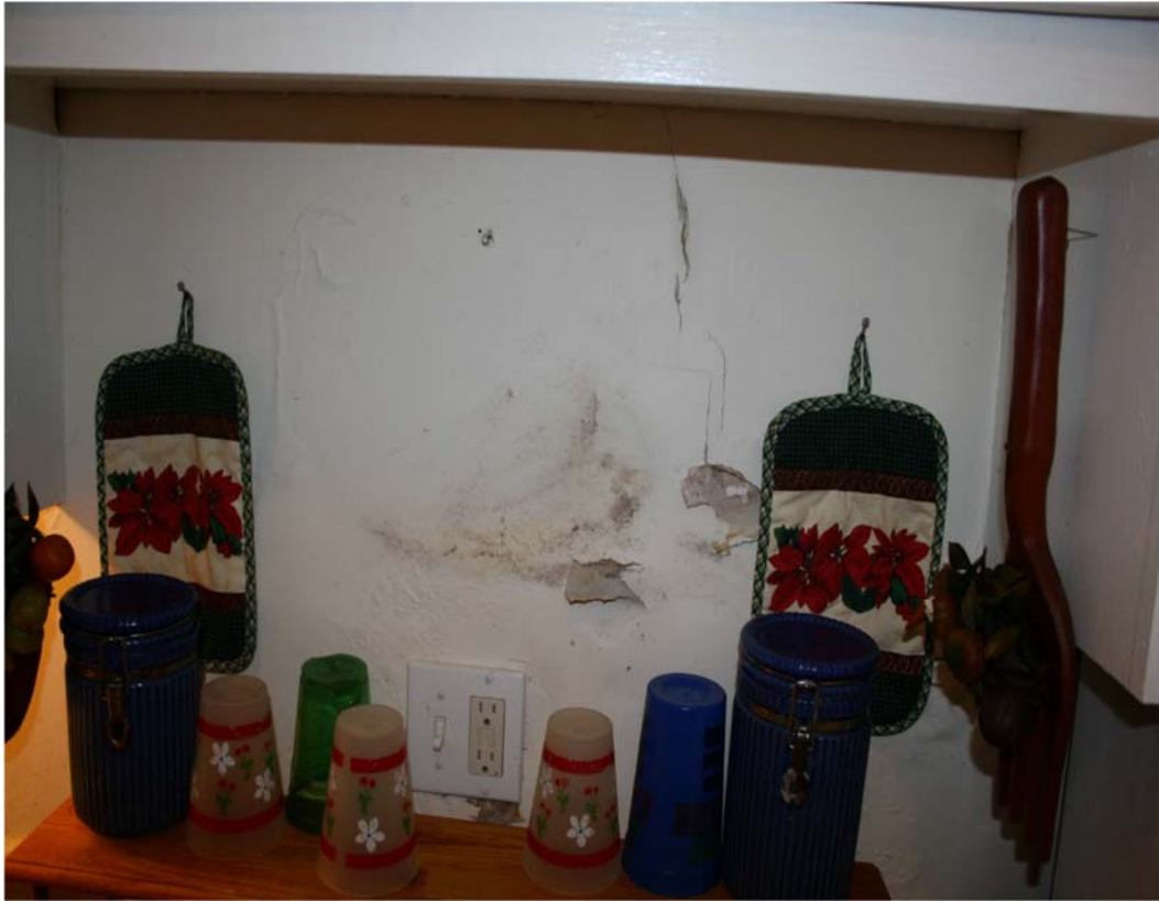
The picture above shows soft drywall from a water leak.
