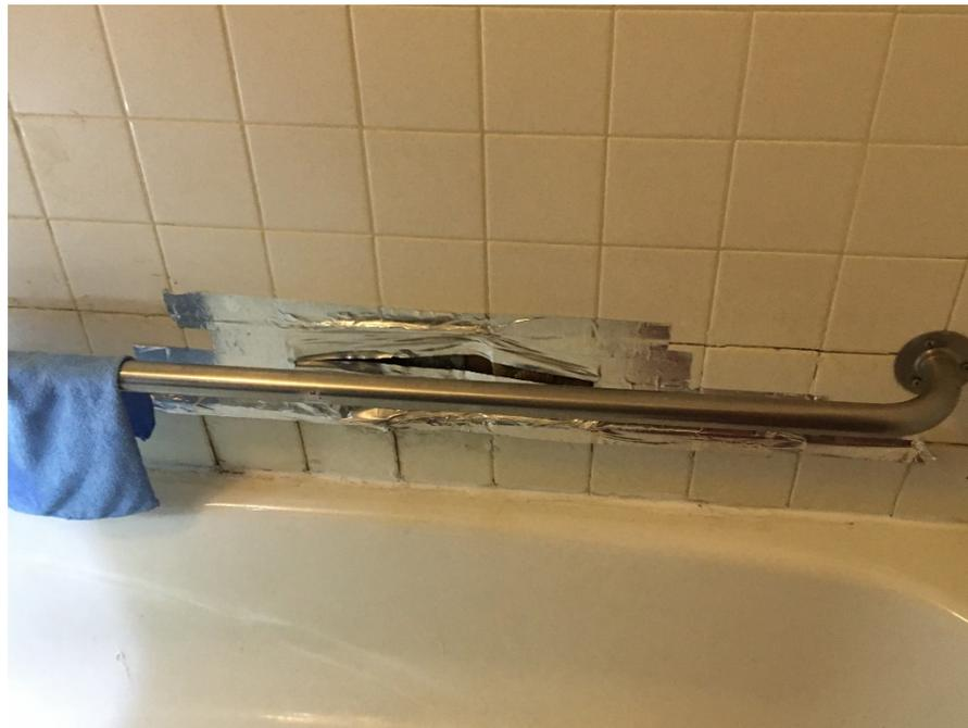
Image 26: Materials not suitable for tile repair - New Rochelle Manor
