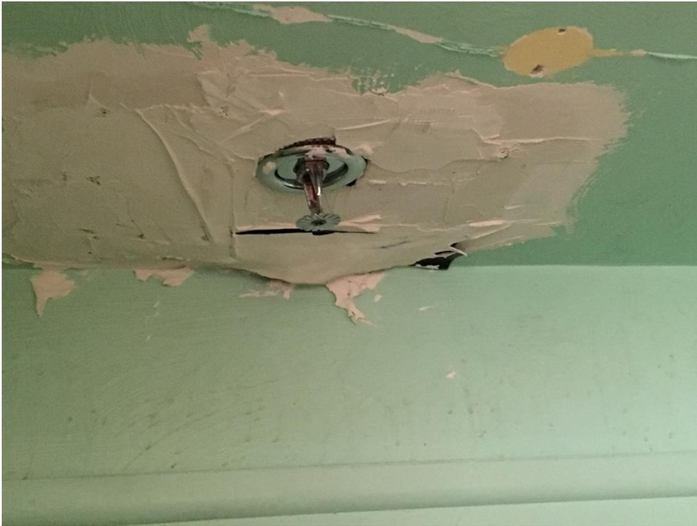
Image 22: Repair not compatible with design and quality of the original and joining decorative materials - Searly Care Center
