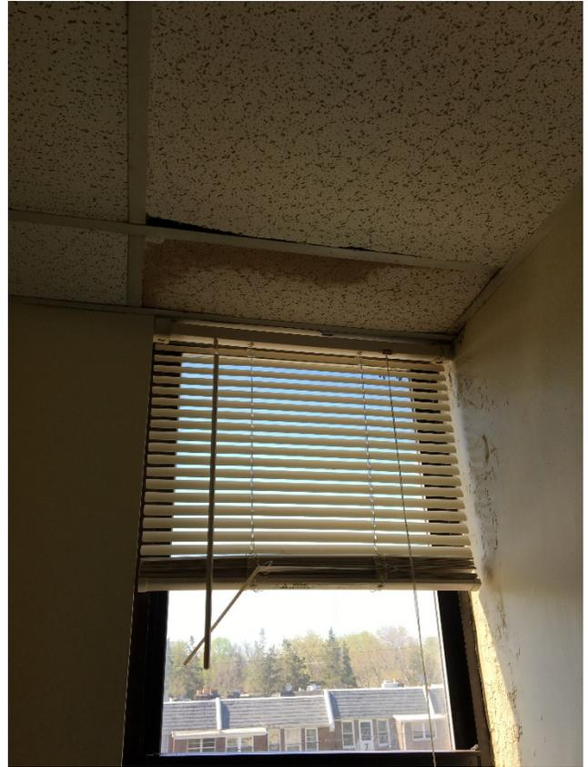
Image 11: Water-stained ceiling tile and water-damaged wall - Bala Nursing Center
