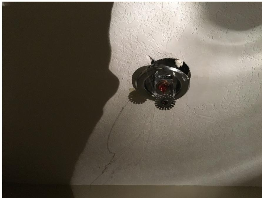
Image 9: Damaged fire sprinkler escutcheon - Cherry Springs Village
