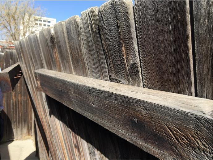
Images 2 and 3: Fencing leaning and sections damaged - Speary Care Center
