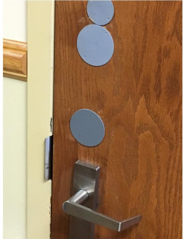
Image 25: Repair not compatible with design and quality of the original and joining decorative materials - Indian River Rehabilitation and Nursing Center
