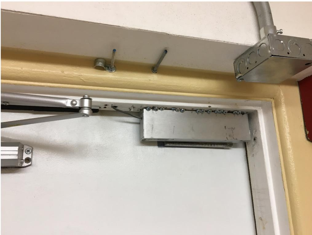
Image 21: Materials not suitable for door magnet repair - Spearly Care Center
