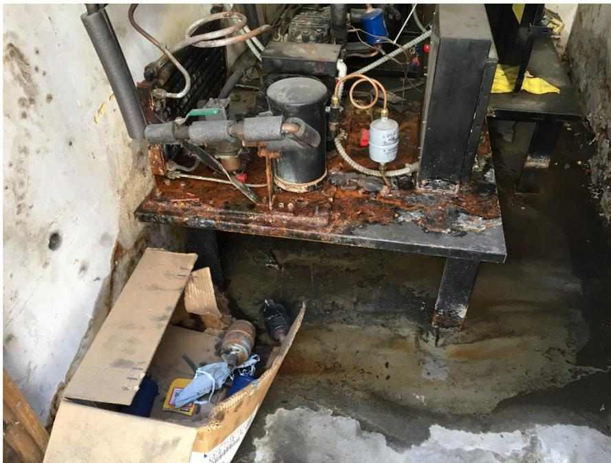
Images 4, 5, and 6: Mold spores and water-damaged refrigeration equipment - Speary Care Center
