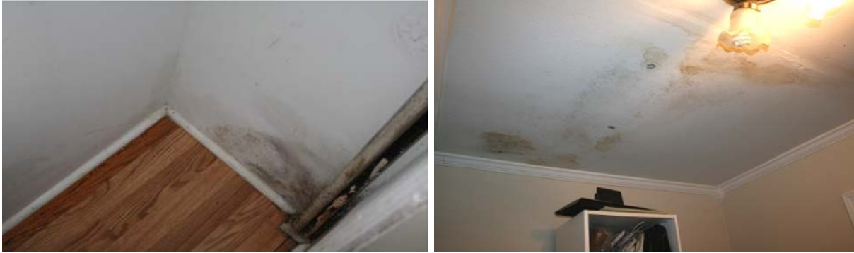
Illustration 3: Mold and mildew identified on newly installed drywall and water damage closet after the roof was repaired
