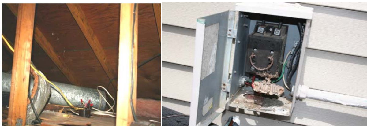
Illustration 2: Electrical splices made outside the junction box and missing interior cover of heating, ventilation, and air conditioning disconnect
