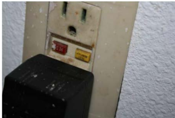
Illustration 1: New ground-fault circuit interrupter not installed
