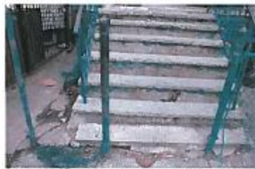
Inspection 29: Deteriorated flooring, posing a falling and tripping hazard with its sharp edges and protruding posts. The Authority did not identify this violation during its November 1, 2017, inspection.
