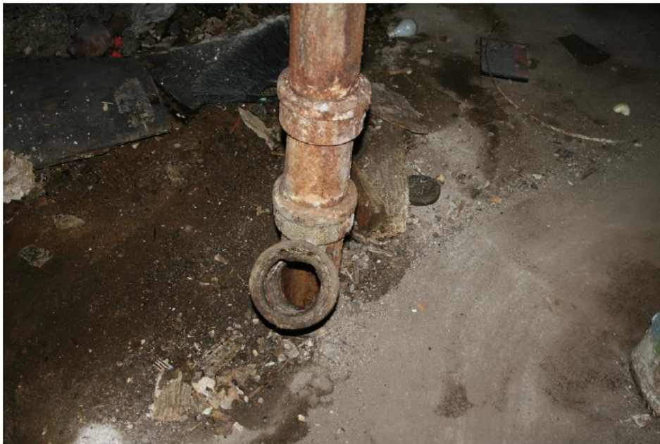
Inspection 9: One of two open sewers in the basement, creating a health hazard because of harmful sewer gases escaping. The Authority did not identify this violation during its December 11, 2017, inspection.
