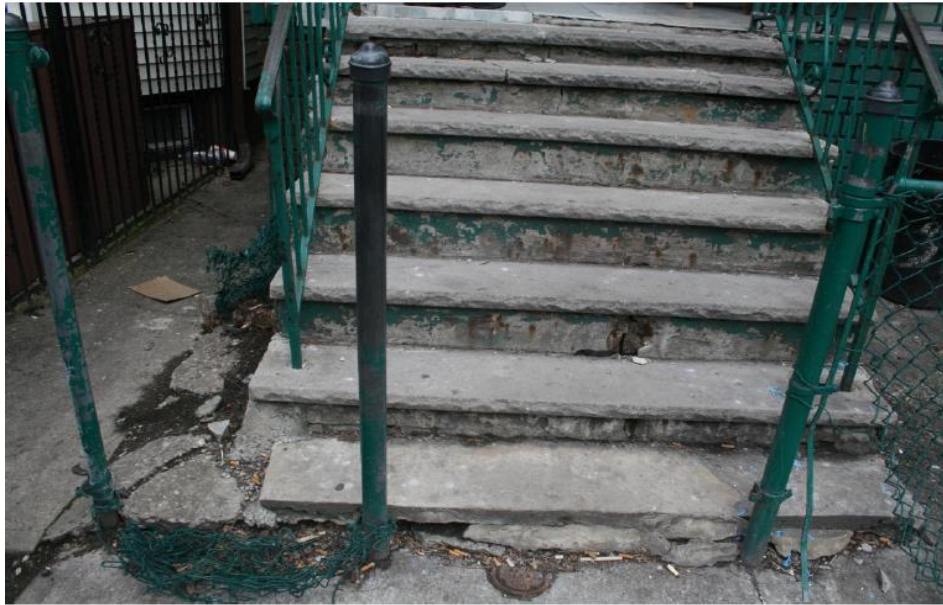
Inspection 29: Deteriorated fencing, posing a cutting and tripping hazard with its sharp edges and protruding posts. The Authority did not identify this violation during its November 2, 2017, inspection.
