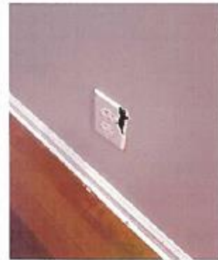
Exhibit 20: Unit 8 Broken outlet cover 170 days after NHA inspection
