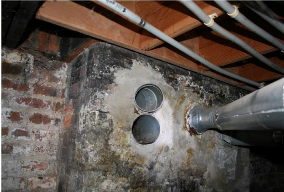
Inspection 15: Open and uncapped flue pipe vents, posing a potential hazard because of carbon monoxide gas seepage. The Authority did not identify this violation during its December 27, 2017, inspection.
