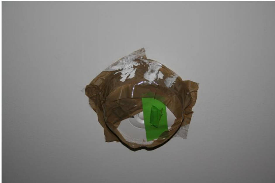
Inspection 2: A taped smoke detector, creating a threat to health and safety. The Authority did not identify this violation during its December 20, 2017, inspection.
