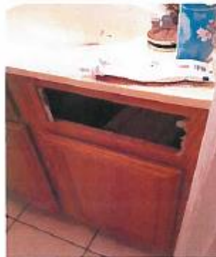
Exhibit 15: Unit 21 Missing vanity panel 156 days after NHA inspection
