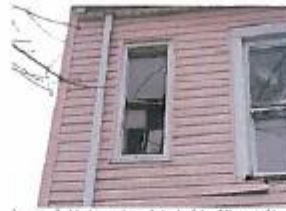
Inspection 1: A broken window with shards of glass falling out of the frame in the kitchen area. The Authority did not identify this violation during its October 23, 2017, inspection.
