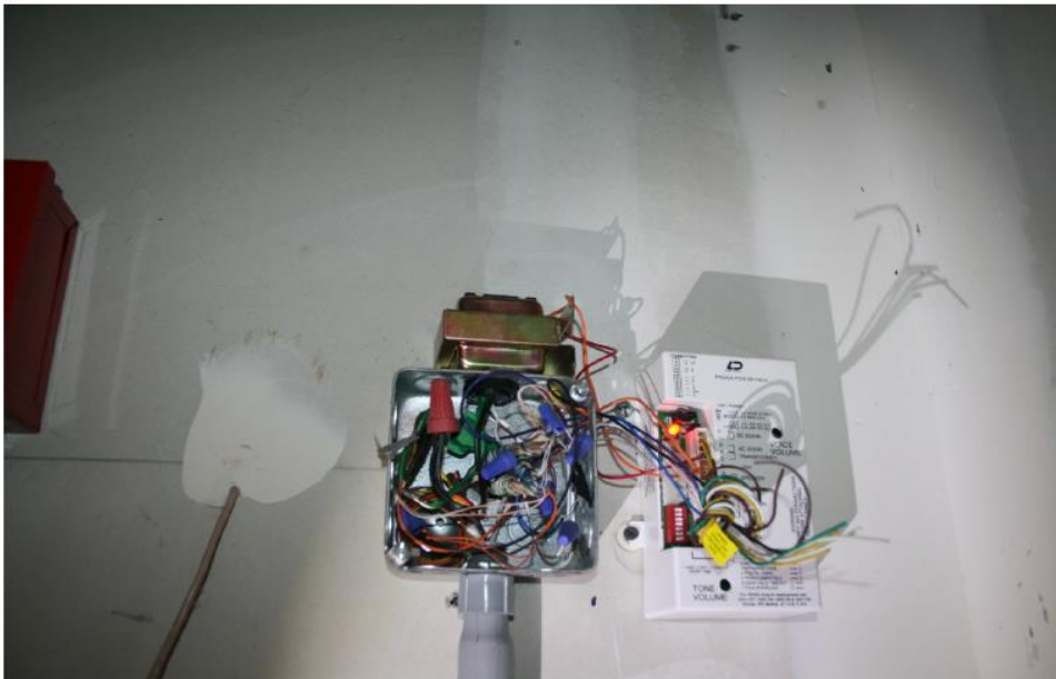
Inspection 24: An open junction box in the first floor sprinkler closet, creating a risk of electrical shock and injury. The Authority did not identify this violation during its October 10, 2017, inspection.
