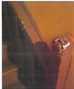
Exhibit 1: Unit 5 There is no HQS requirement for a handrail be fully graspable
