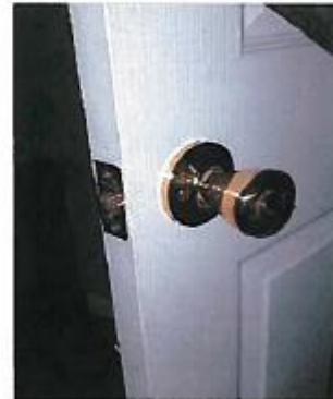
Exhibit 7: Unit 25 Single keyed lock with thumb turn
