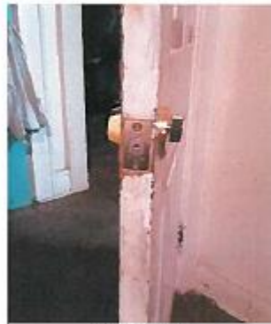
Exhibit 6: Unit 24 Single keyed lock with thumb turn
