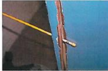
Inspection 25: A cracked rear entry door jamb, posing a threat to space and security. The Authority did not identify this violation during its November 2, 2017, inspection.
