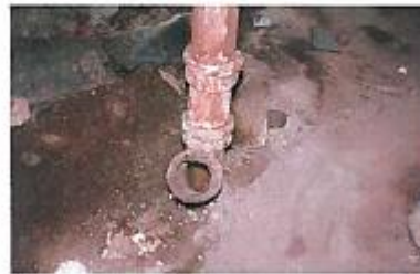
Inspection 2: One of two open sewers in the basement, creating a health hazard because of harmful sewer gases escaping. The Authority did not identify this violation during its December 11, 2017, inspection.
