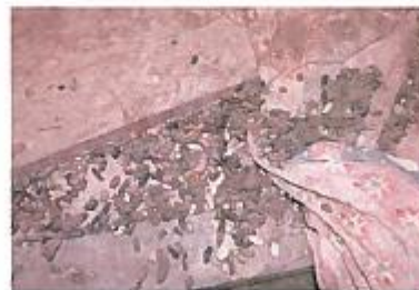
Inspection 7: Excessive rat droppings in the bathroom, indicating a heavy rodent infestation and creating an unsanitary condition for the tenants. The Authority did not identify this violation during its October 23, 2017, inspection.
