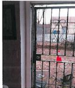
Exhibit 12: Unit 22 Back door locked 119 days after NMA inspection
