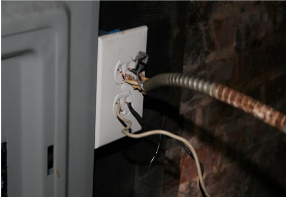
Inspection 9: Boot-legged wiring in the basement, creating a potential fire hazard and threat to health and safety. The Authority did not identify this violation during its December 11, 2017, inspection.
