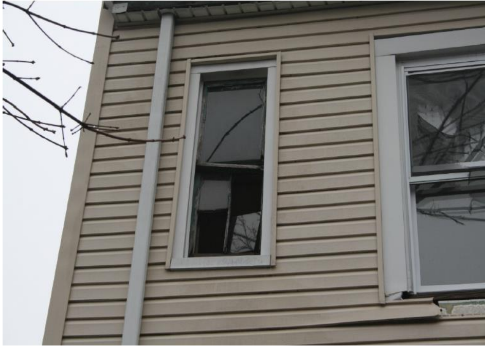
Inspection 7: A broken window with shards of glass falling out of the frame in the kitchen pantry. The Authority did not identify this violation during its October 23, 2017, inspection.
