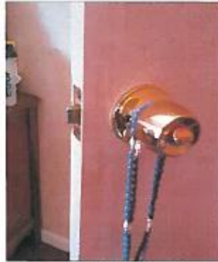
Exhibit 8: Unit 15 Single keyed lock with thumb turn
