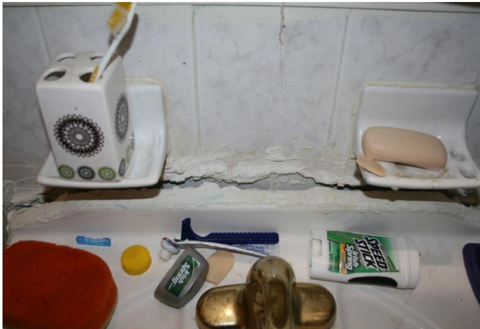
Inspection 9: A detached wash basin and cabinet, creating an unhealthy sanitary facility. The Authority did not identify this violation during its December 11, 2017, inspection.
