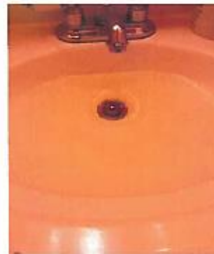
Exhibit 16: Unit 19 Slow sink drain 140 days after NHA inspection
