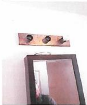
Exhibit 17: Unit 11 Missing light bulbs 166 days after NHA inspection
