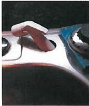
Exhibit 13: Unit 16 Missing sprayer collar 153 days after NHA inspection
