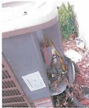
Exhibit 19: 912 Longworth St Open AC compressor compartment 166 days after NHA inspection
