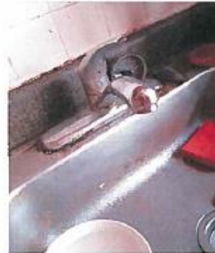
Exhibit 14: Unit 17 Rust on kitchen faucet 152 days after NHA inspection
