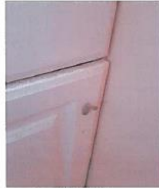
Exhibit 22: Unit 5 Broken cabinet handle 175 days after NHA inspection
