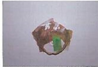
Inspection 2: A taped smoke detector, creating a hazard to health and safety. The Authority did not identify this violation during its December 20, 2017, inspection.
