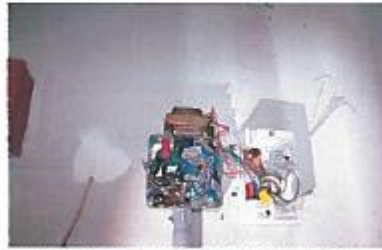
Inspection 24: An open junction box in the first floor stairwells closes creating a risk of electrical shock and injury. The Authority did not identify this violation during its October 10, 2017, inspection.
