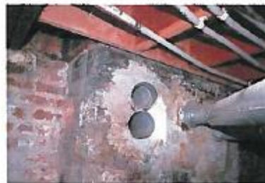
Inspection 15: Open and uncapped fire pipe vents, posing a potential hazard because of carbon monoxide gas leakage. The Authority did not identify this violation during its December 27, 2017, inspection.
