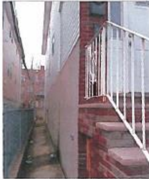
Exhibit 21: Unit 11 Missing downspout section 166 days after NHA inspection
