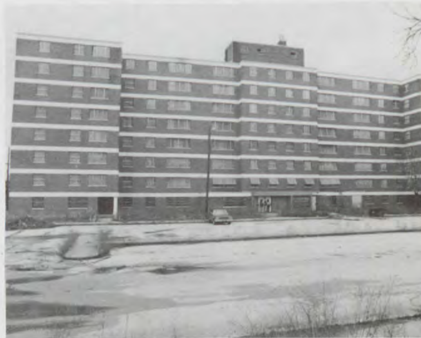
One of two boarded-up and uninhabited buildings on which a $2.2 million contract was awarded, $1.4 million was disbursed to the contractor, and only $150,000 worth of work was performed.
