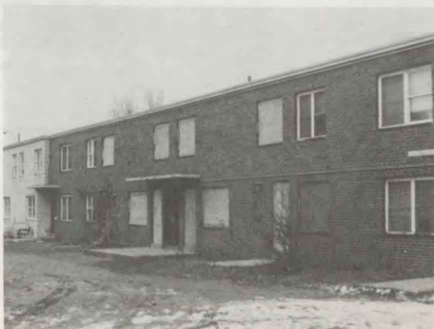
Examples of CMHA units boarded up for long periods of time because of inadequate maintenance program.
