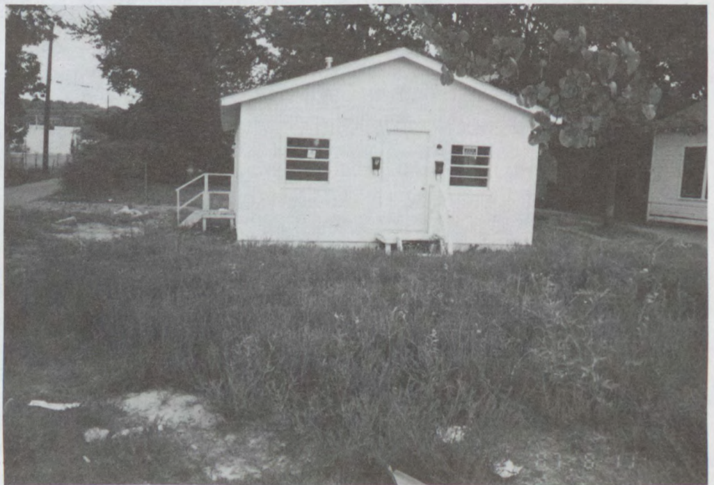
Newly constructed unit after original unit burned in North Little Rock. Owner collected $34,000 in insurance proceeds, exceeding the $29,560 documented owner costs for the project.
