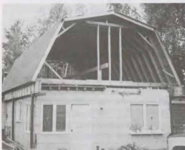
1992 photo of work certified completed in 1989
