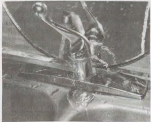
Kitchen sink faucet that will not turn water off.
