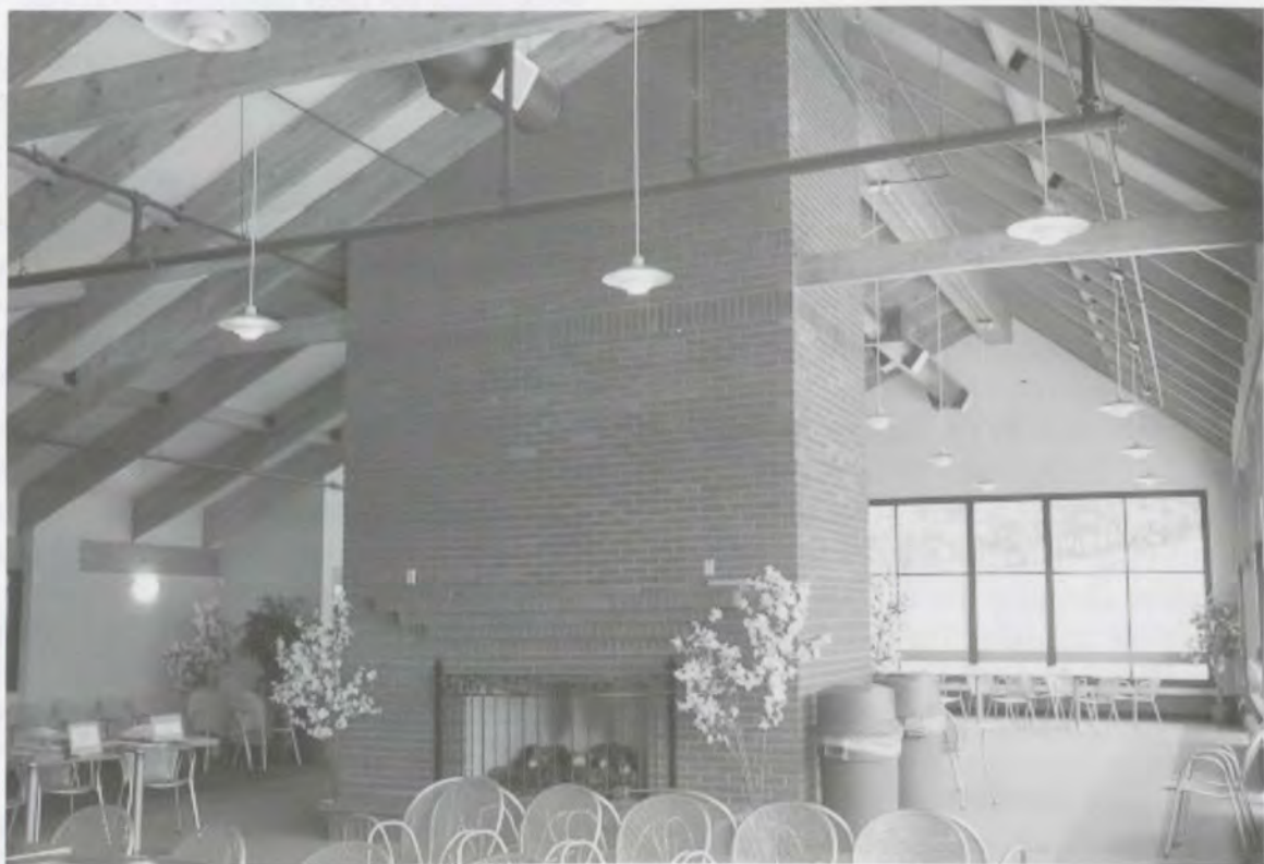
Ski chalet at Parkway Recreation Center Project in Utica, NY. Renovated with CDBG Funds.
