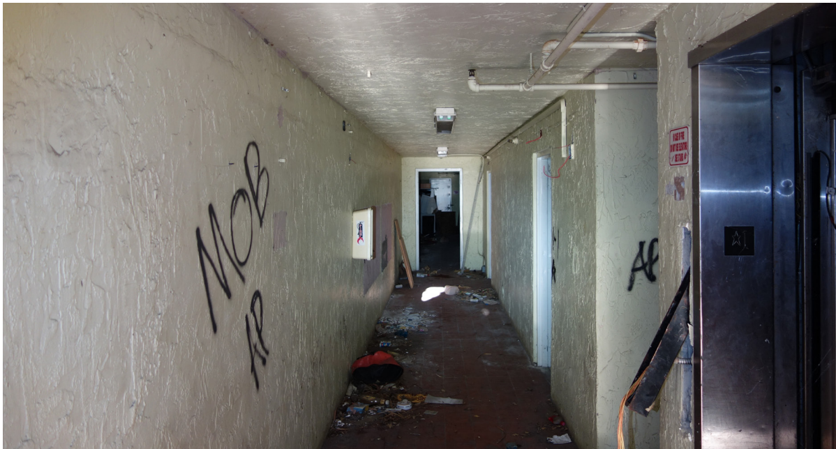
Interior hallway showing the state of disrepair
