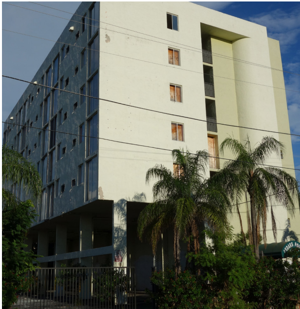
Exterior of Cedars Pointe complex in state of disrepair
