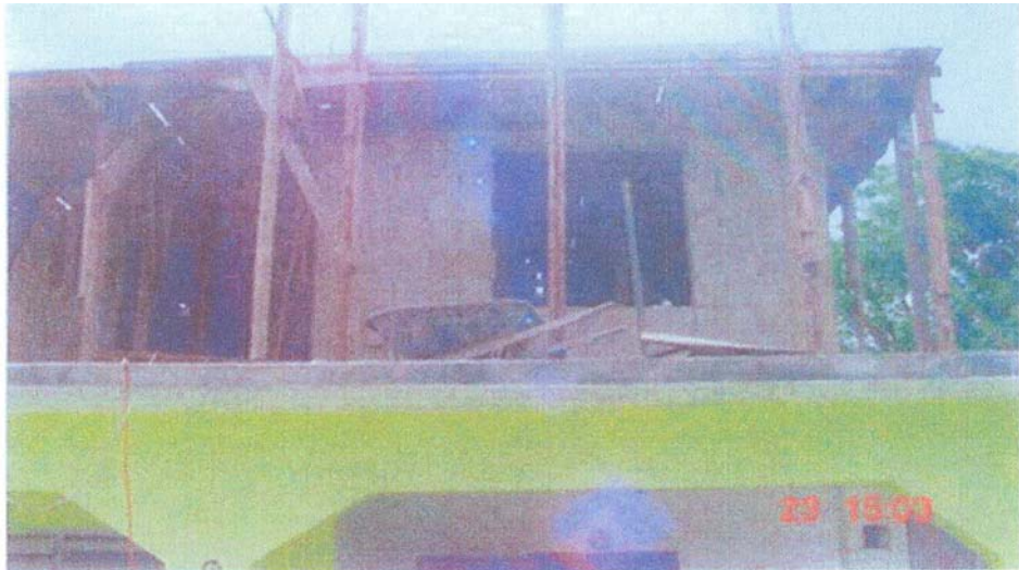
Figure 6: Case Number 2002-099- Before Rehab
