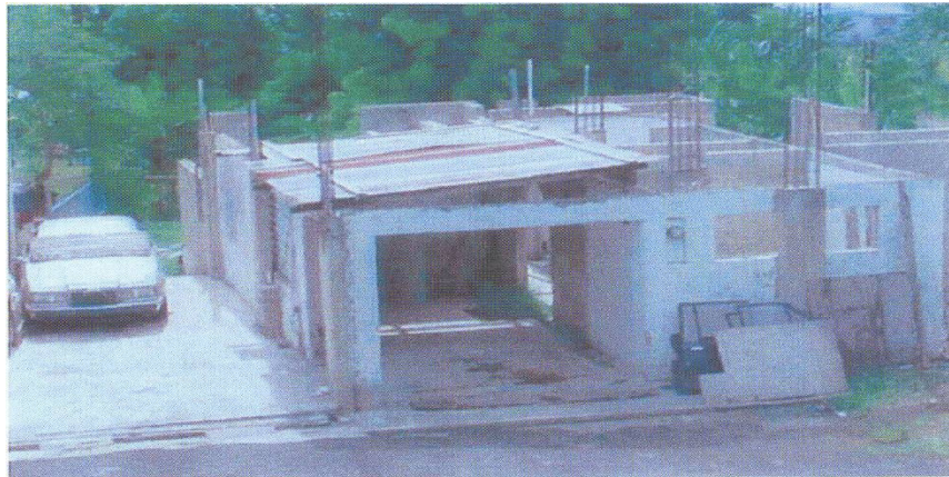
Figure 8: Case Number 2000-587 Before rehab
