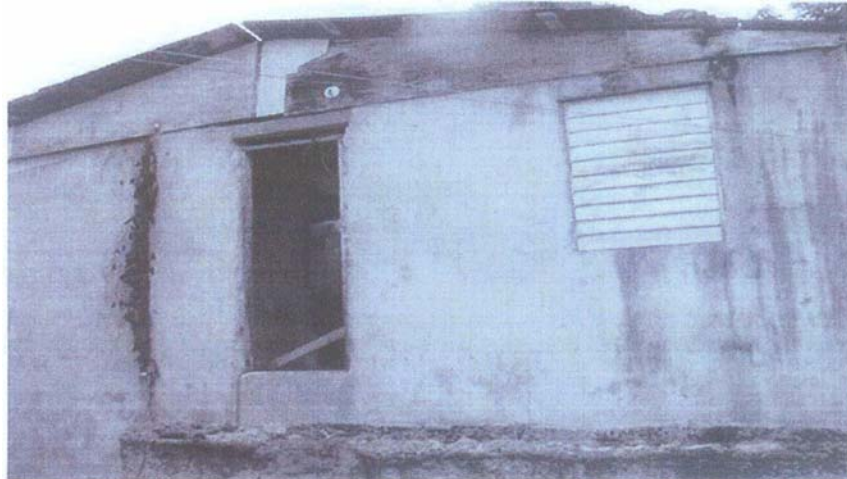
Figure 4: Case Number 2000-607- Before Rehab
