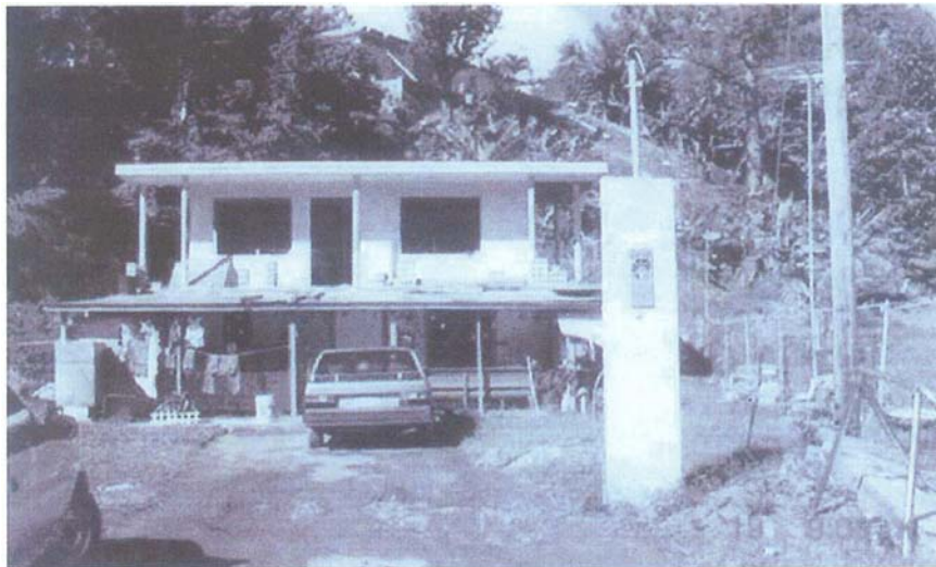
Figure 2: Case Number 2004-003 photo before the rehabilitation
