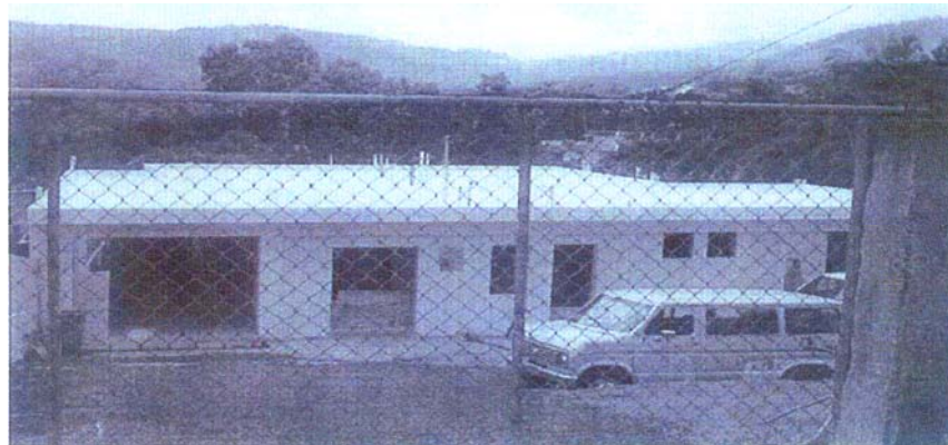
Figure 9: Case Number 2000-587 after work performed
