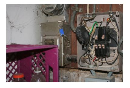
Inspection #24: The cover was missing on the metal security box, and the electrical wiring was exposed.
