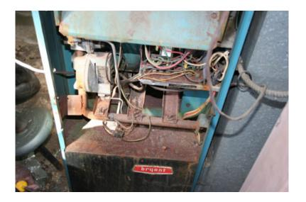
Inspection #43: The heating system's metal casing was corroded, and metal was fatigued (pitted) due to long-term use.
