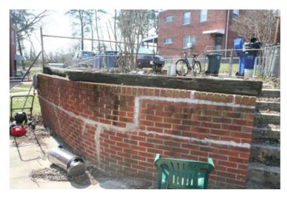
Inspection #19: The required handrail was missing on the stairs.
