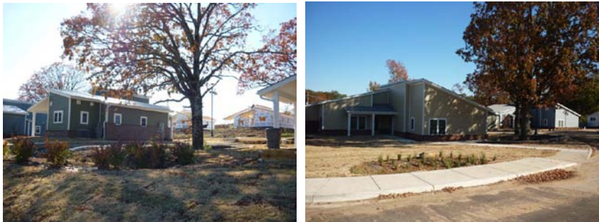
Legacy Homes at Granite Mountain Senior Housing ARRA Funded Project
