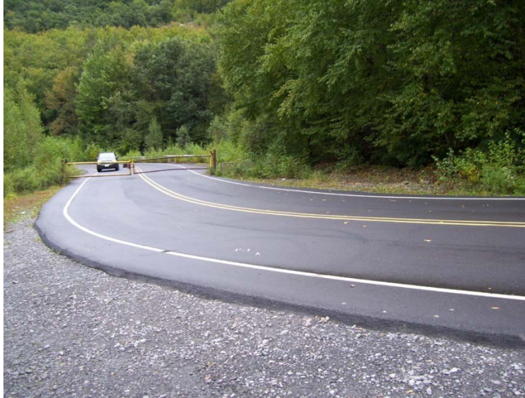
Earth Conservancy street improvements (completed)
