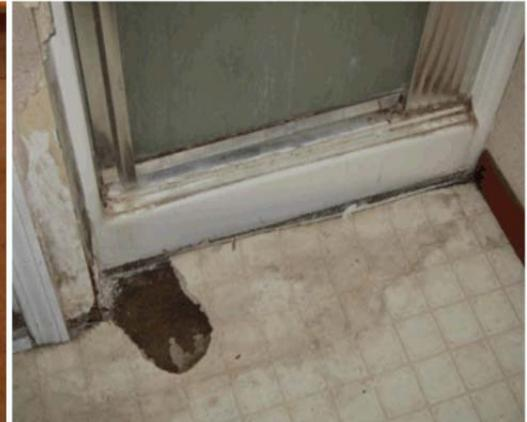
The paint was peeling, and the vinyl was torn in this bathroom. According to a worksheet provided by the compliance department, some of these houses had lead-based paint.
