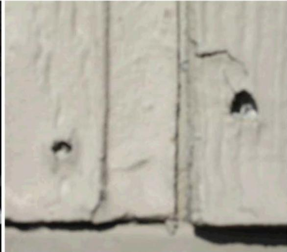
The siding was not properly prepared before being painted, which caused it to continue to deteriorate.
