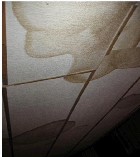
The ceiling tiles showed significant water damage but had not been replaced.
