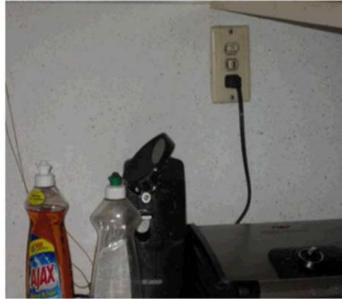
Electrical outlets were not always updated. There were no ground wires or ground fault circuit interrupters in several houses.
