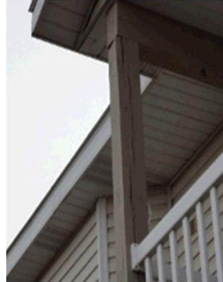
Another deck post was cracked where the railing was attached.
