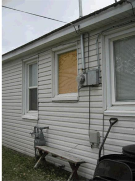
The window was removed, but the siding was not repaired.
