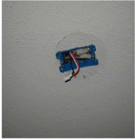
A hard-wired smoke detector was missing, leaving exposed electrical wires.
