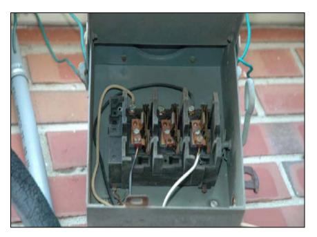
Client Identification #014689: The power line and junction box were loose.
