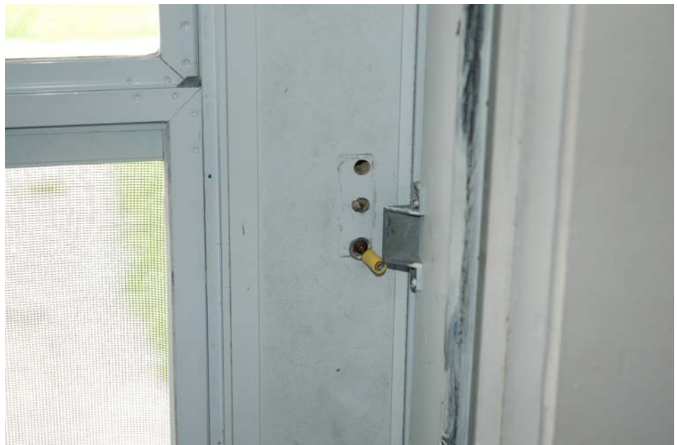
Unit #35: Broken/missing latch on front storm door.
