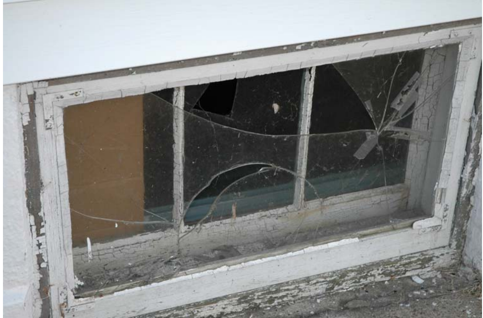
Unit #33: Broken glass pane on the basement window.
