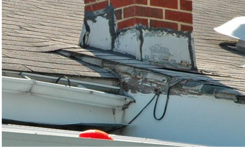
Inspection #46: The roof failed next to the chimney in back of the house. The roof settled approximately 5" near the chimney. This violation was not identified during the Authority's December 13, 2007, inspection.
