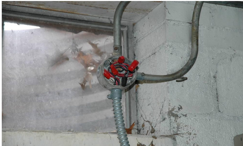
Inspection #47: The cover plate is missing from the junction box on a wall in the common laundry room .
