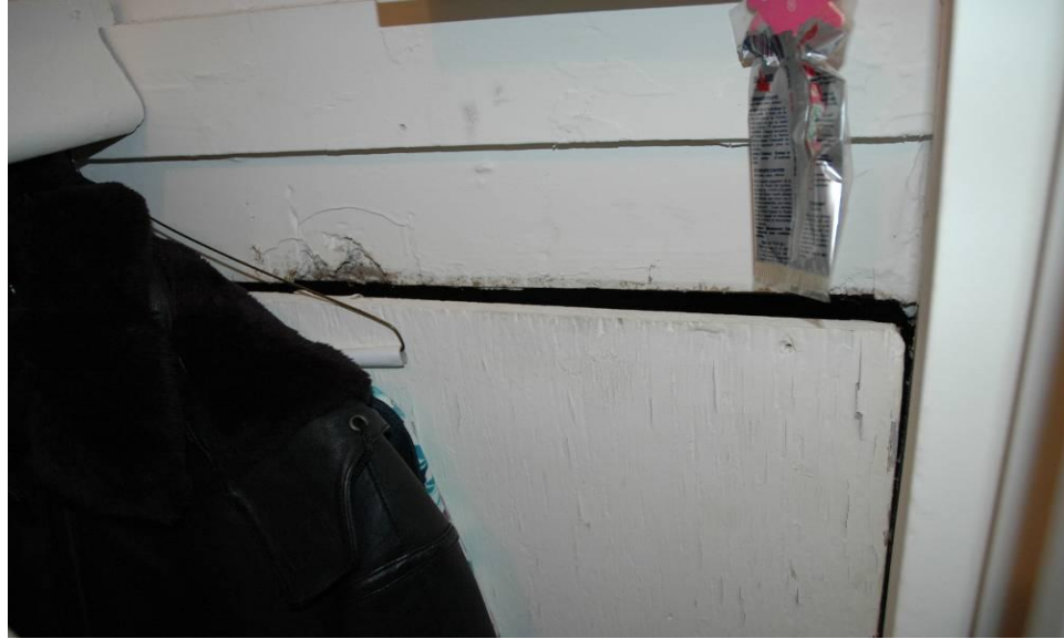
Inspection #33: The plywood panel inside the right/rear bedroom closet separating the closet from a gas-burning heating furnace is not secured. Combustible items are stored against the plywood panel. This violation was not identified during the Authority's December 20, 2007, inspection.
