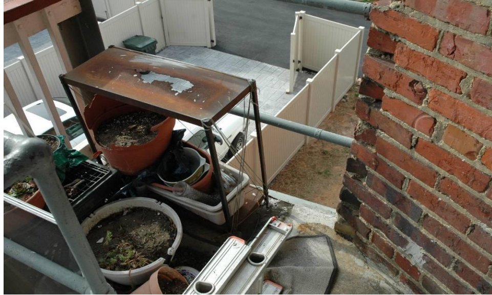
Inspection #8: Planters and other small objects are stored on the balcony without a curb to keep them from falling three stories onto a sidewalk. This violation was not identified during the Authority's November 1, 2007, inspection.
