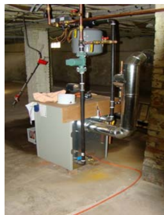
Figure 2 - New heating equipment
