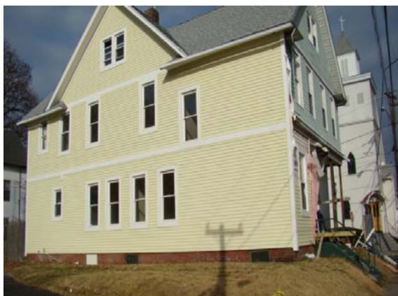
Figure 1 - New exterior siding
