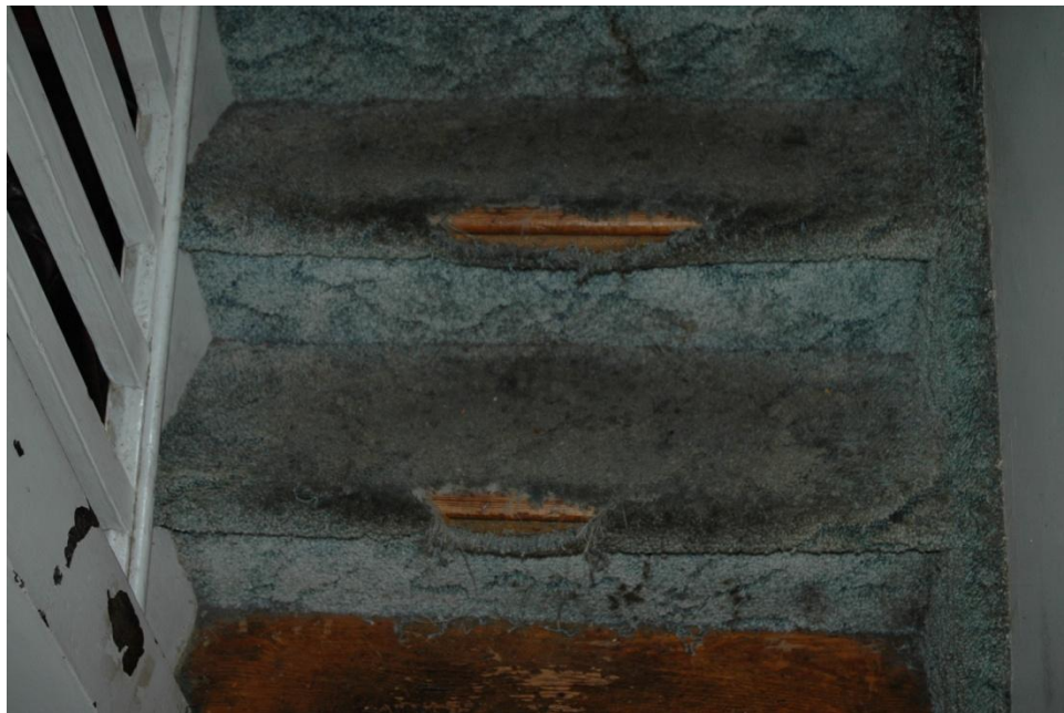
Inspection #24: The carpet is torn on the stairway to the second floor.
