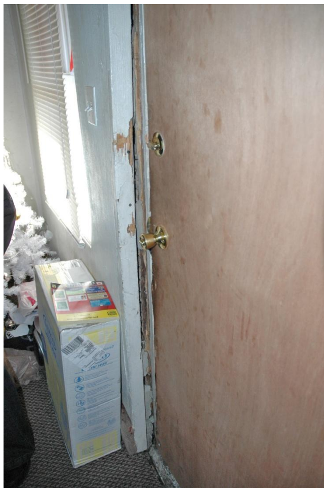
Inspection #72: The front entrance doorway has a large vertical gap along the entire height of the door jamb and the wall.
