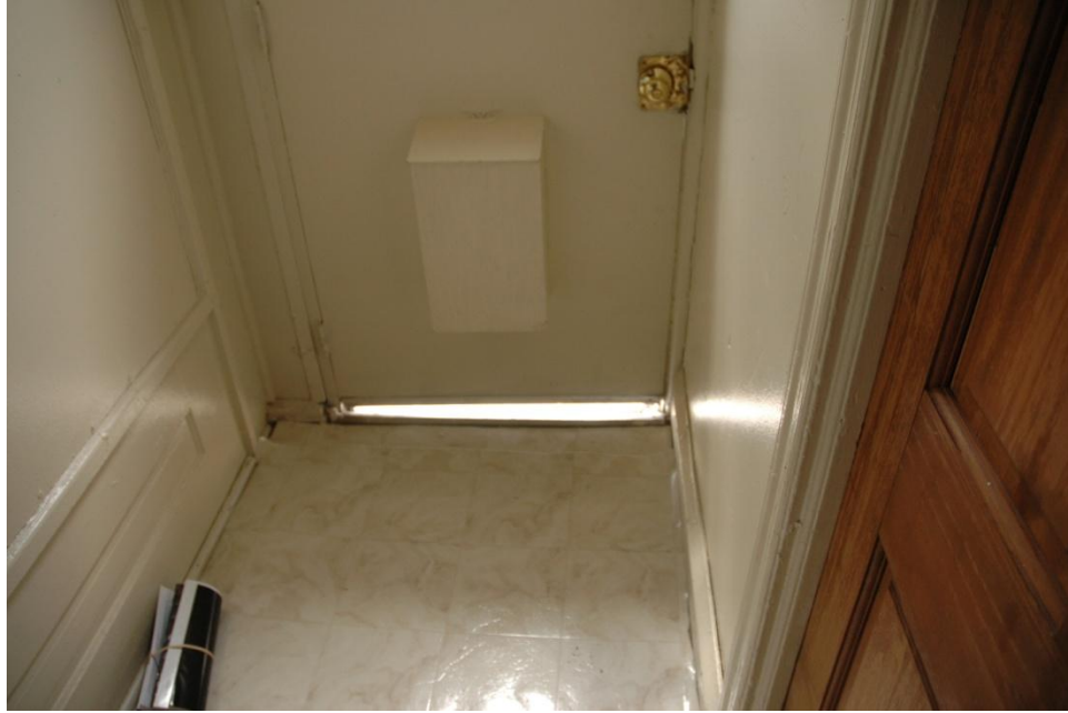
Inspection #30: A gap under the front entrance door allows air infiltration and vermin to enter the unit.
