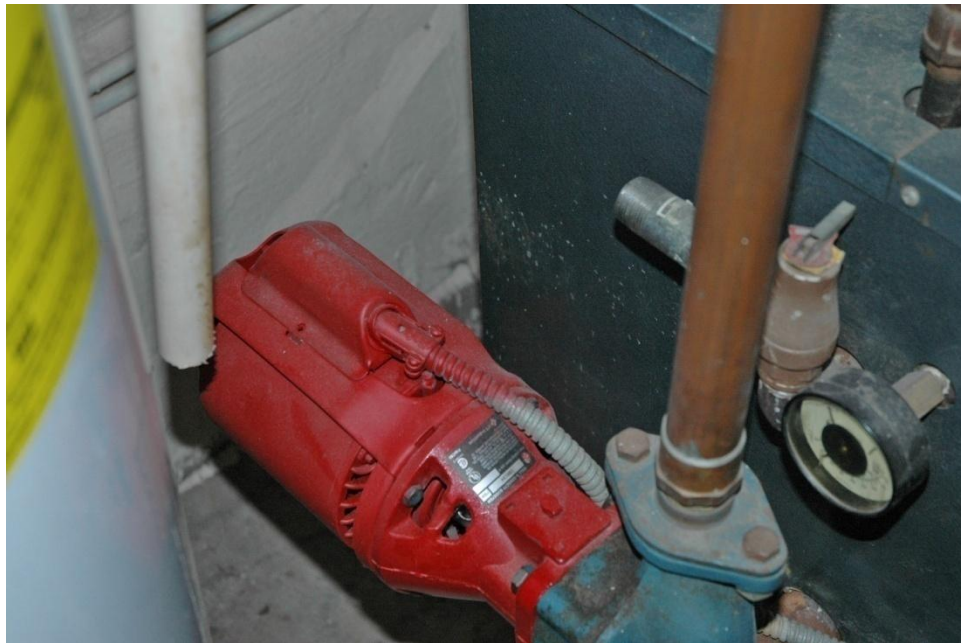
Inspection #35: The water heater discharge pipe (left) is too short and the boiler discharge pipe (right) is horizontal.
