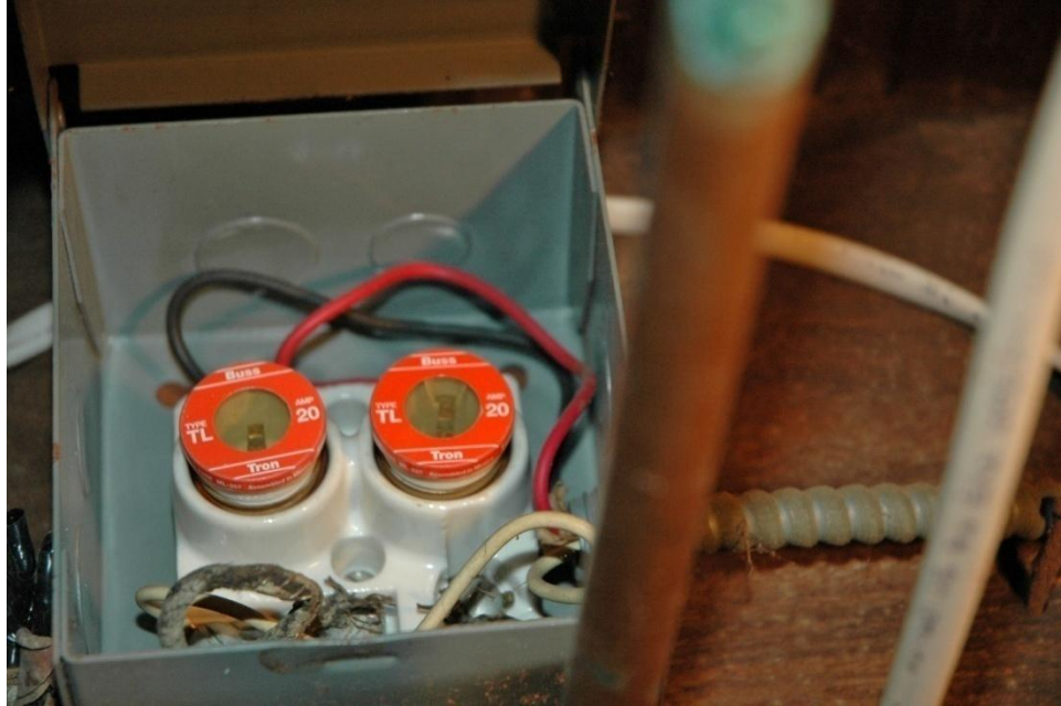
Inspection #70: The fuse box is unsecured and missing its internal cover, exposing electric contacts.
