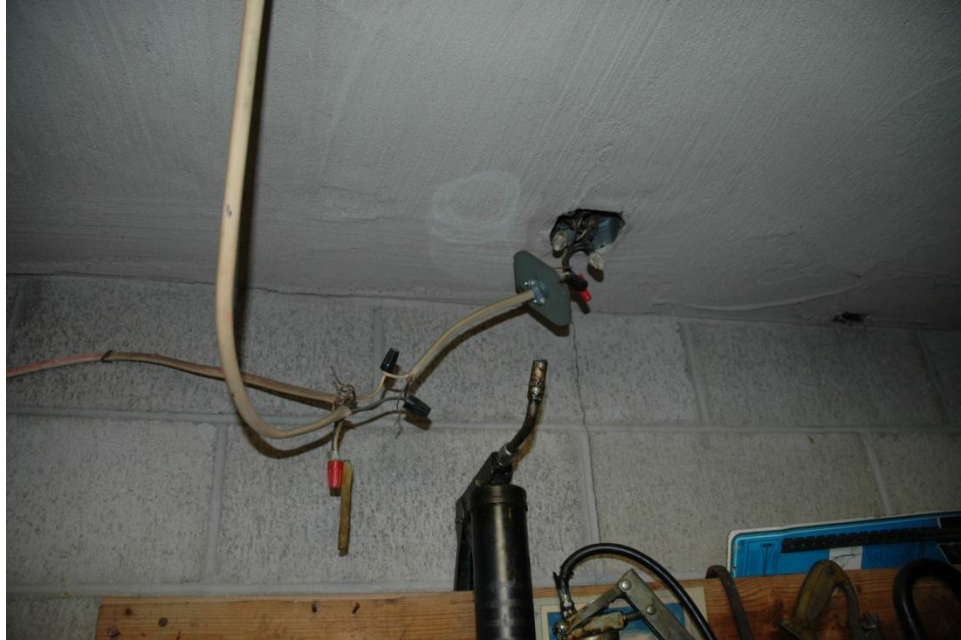
Inspection #25: There is a loose cover on a junction box, and wires are spliced outside a junction box.
