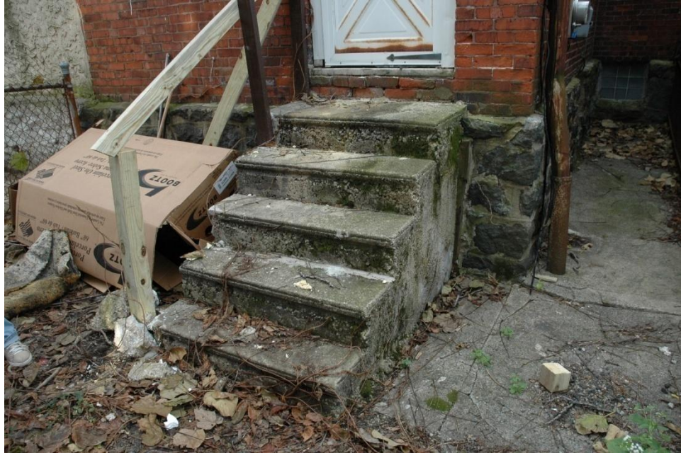
Inspection #11: The open side of the rear stairway needs a guardrail.
