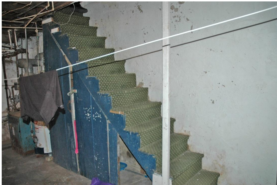
Inspection #36: The stairway to the basement requires a handrail. The stairway requires a guardrail on the open side.
