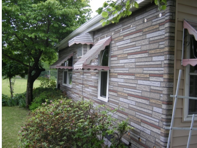
Vinyl siding was not installed around the entire house in project #1843.
