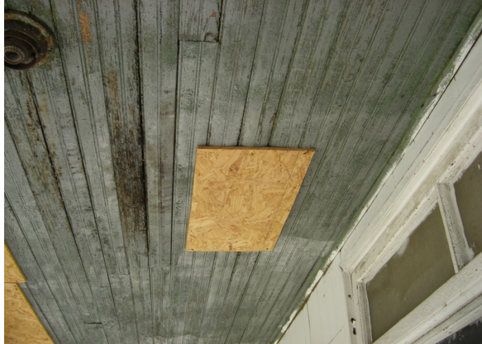
Strips of oriented strand board were screwed to the front porch ceiling of project #1832.
