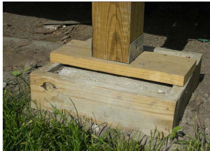
For project #1832, the contractor straddled boards from one side of the pier formwork to the other and rested the columns on the boards instead of on the front porch's concrete piers.
