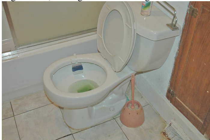
A nonhandicapped toilet and no grab bar were installed in project #1714.
