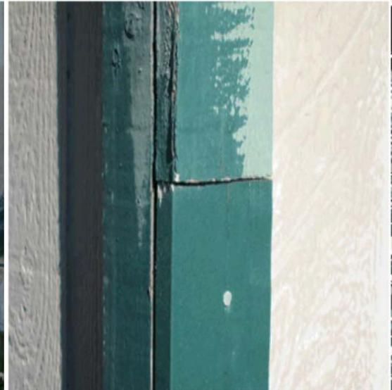
Repairs were made, but the seams were not caulked, and the painting was not completed.
