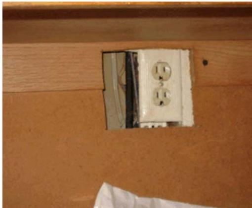
A hole was cut larger than the electrical box, leaving exposed electrical wires.
