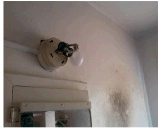
There were missing light fixtures in several of the units. In addition, some of the bathroom fans did not work.
