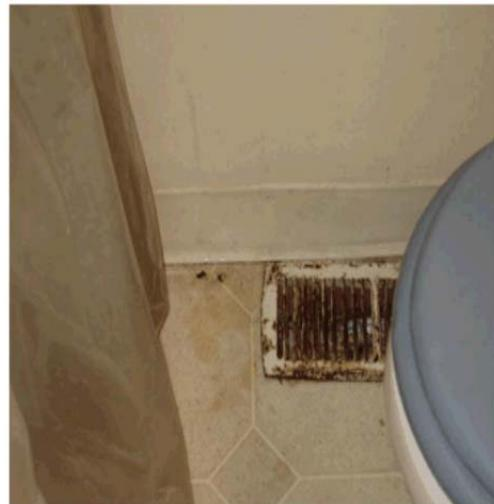
The heating vent was extremely rusted but had not been replaced.
