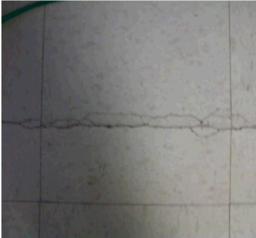
Commercial tile floors were cracking in most of the units inspected. The property manager stated that when some of the tiles were replaced, dirt was found under them.
