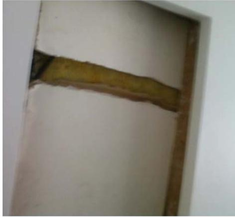
The attic access cover was broken in several of the units, leaving the insulation exposed.
