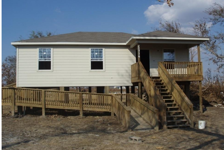
Elevation project, Sabine Pass, Texas – Although the area flooded, the home was not damaged because it was elevated.
