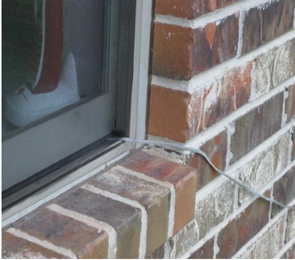
Picture 1: Occupied unit – screen cut and a phone cord inserted through the screen
