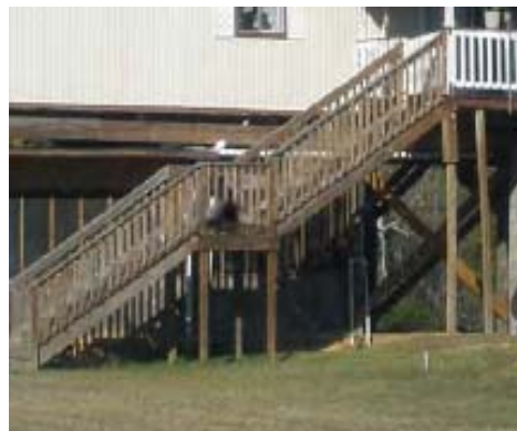
As a comparison, this home underwent elevation construction.
