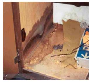
Moisture damaged drywall at window frame at Saraland Manor Apartments. The age and condition of window units makes them too difficult to operate and subject to moisture intrusion.
