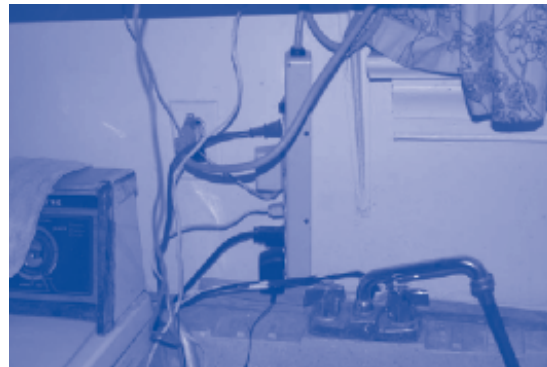
Power strip connected to an ungrounded receptacle near sink in unit located at 3813 Kellar.
