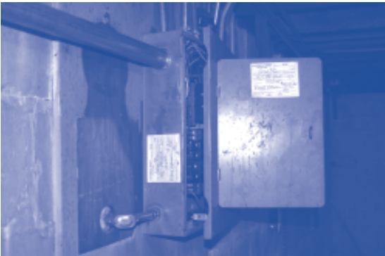
3960 Maryland: Cover on electric panel not securely fastened; panel also missing a breaker.
