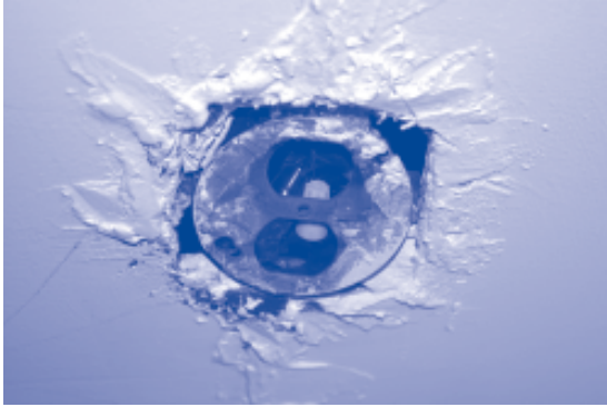
3837 Maryland: Exposed wires in basement junction box.
