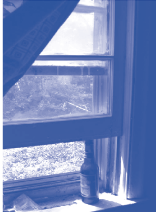
Window has no counterweights and does not stay up. Bottle keeps window propped up for the unit located at 3905 Proctor.
