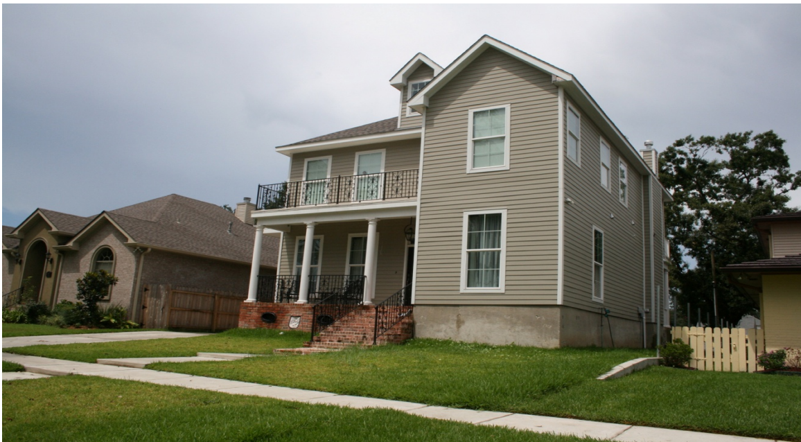
6628 General Diaz Street, New Orleans, LA (East Bank, Lakeview District)
